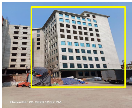
Building No. 06 (New Building)
