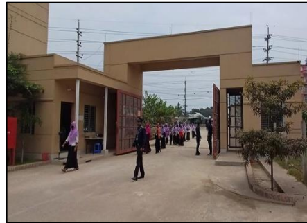
Diesel Store and Security Building
