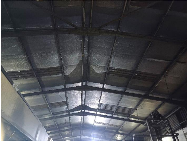
Dyeing shed-2 (Main Part Steel)
