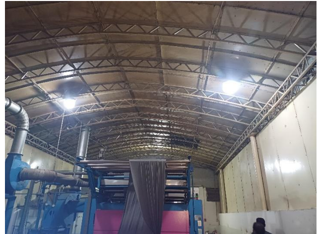
Dyeing shed-2 (Extension Part Steel)
