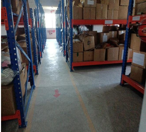
Racks without anchorage
