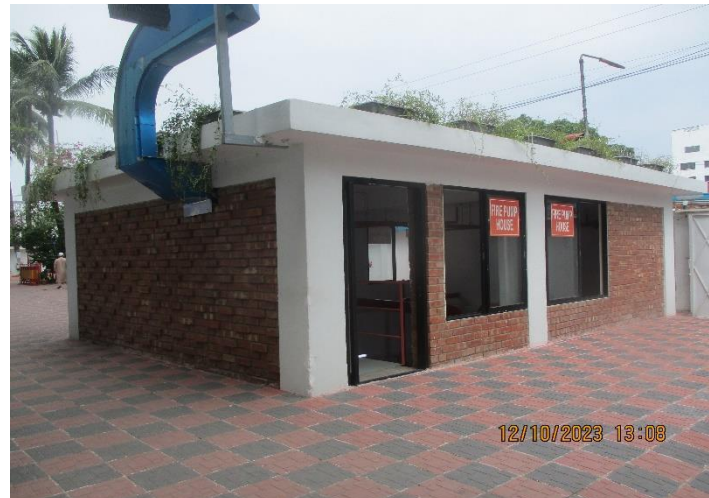
Fire Hydrant Pump Room
