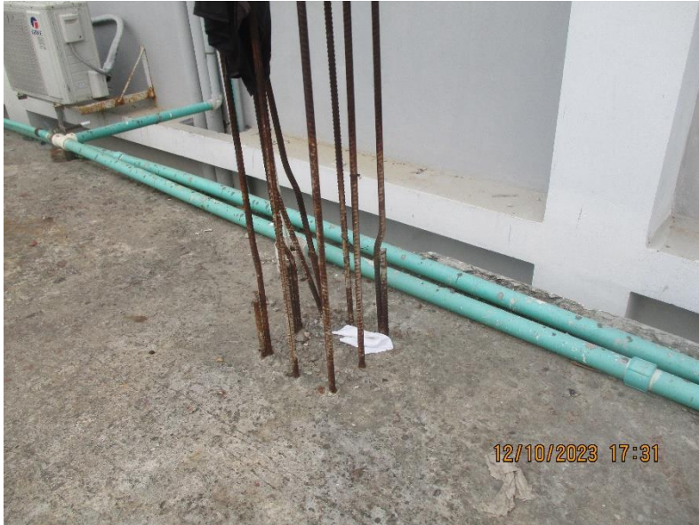
Exposed rebar on roof
