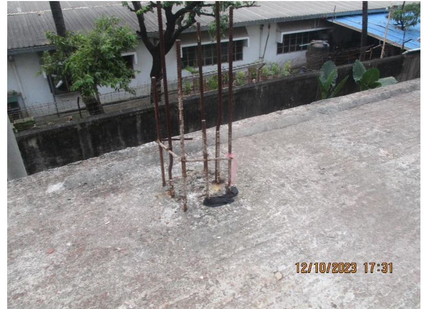
Exposed rebar on roof
