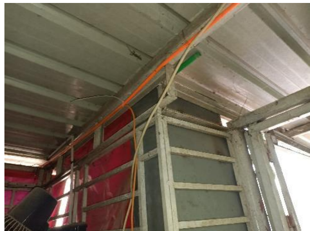
Framing of Idle Machine Shed
