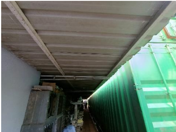
Idle Machine Shed
