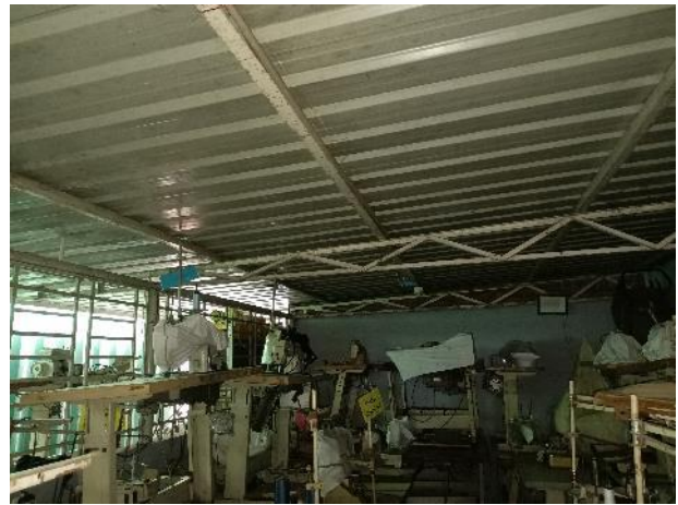
Framing of Idle Machine Shed
