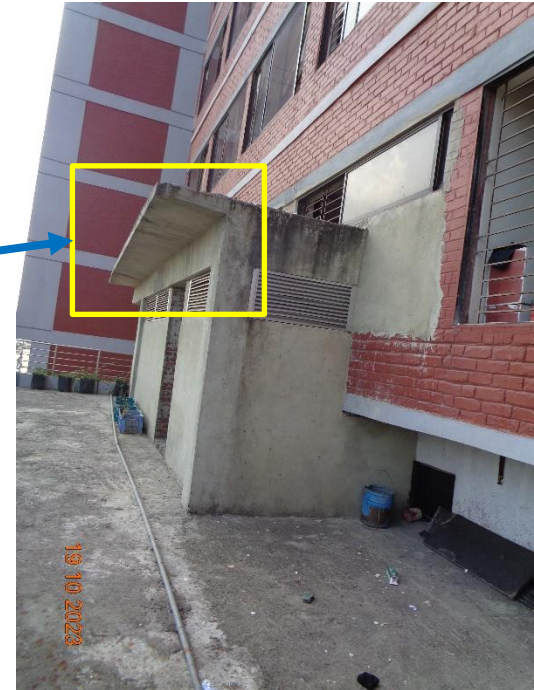
Marked beams layout not matched with on-site condition
