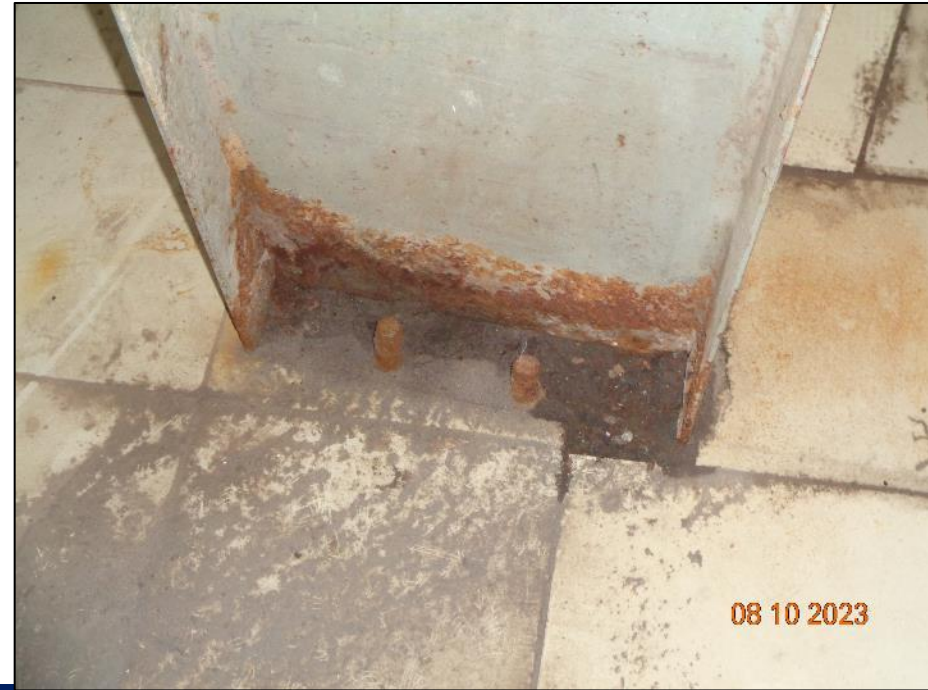
Corrosion in steel section
