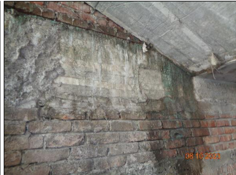
Signage of water ponding at roof, dampness at beam & wall
