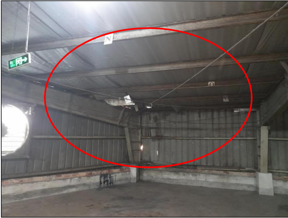
Loose cable bracing (Finishing & Warehouse Shed )
