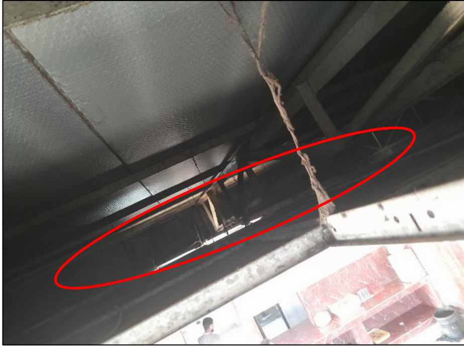
Purlin inserted to brick wall
