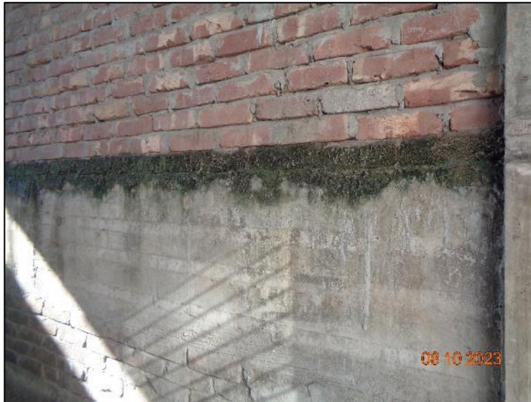
Signage of water ponding at roof, dampness at beam & wall
