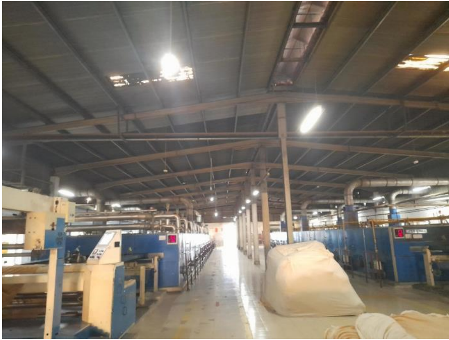
Portal frame along short direction.
