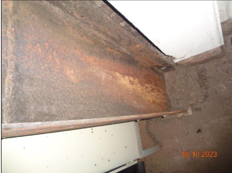
Corrosion in steel section
