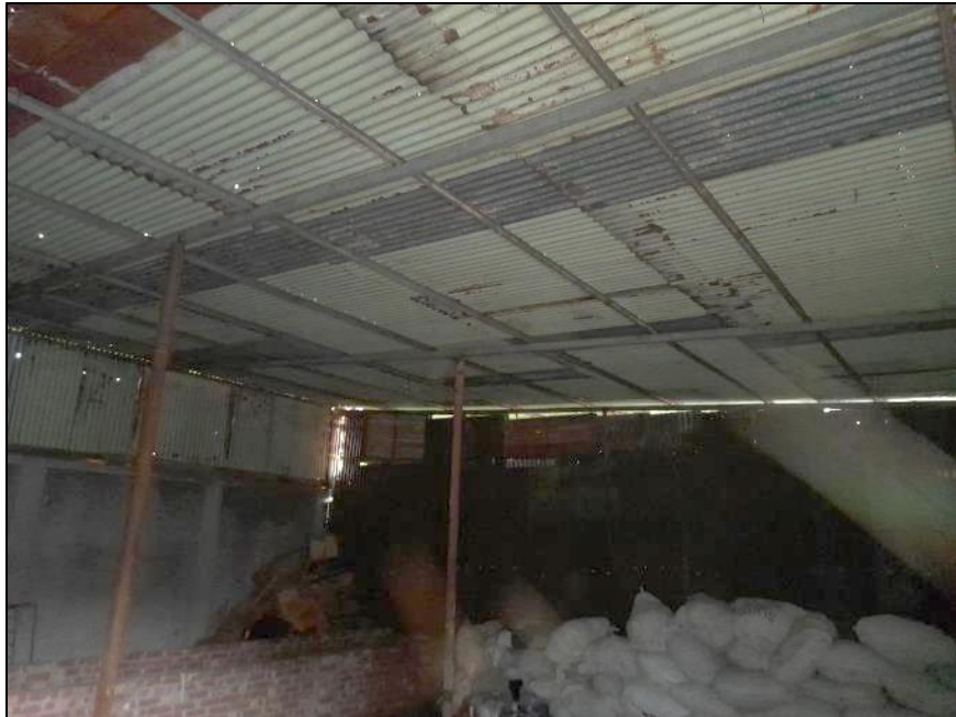
Poor connection between steel members
