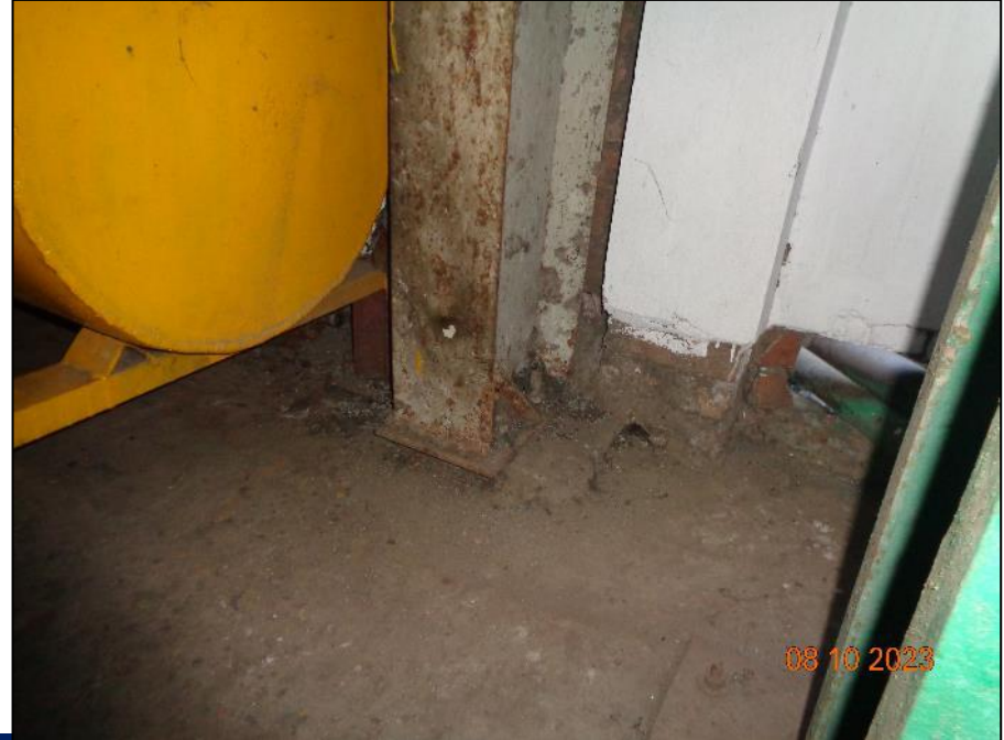
Corrosion in steel section
