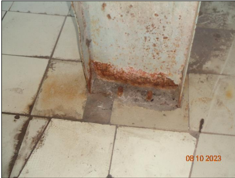
Corrosion in steel section
