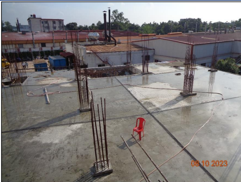
Extension work was found ongoing
