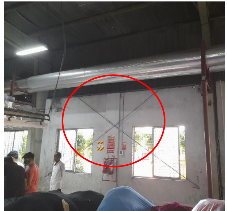
Loose cable bracing (Finishing & Warehouse Shed )
