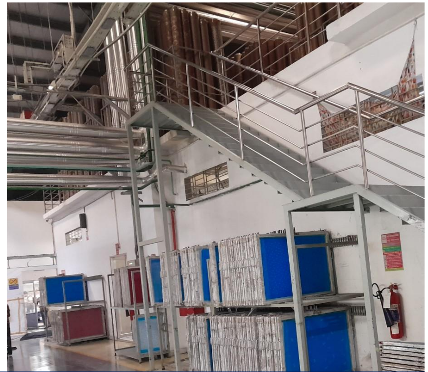
Mezzanine floor having no load plan
