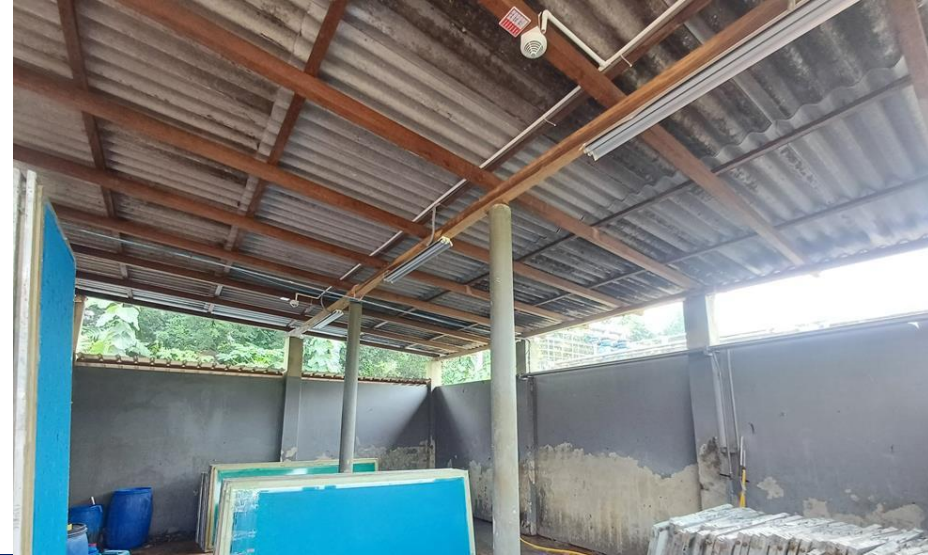
Apparently non-engineered structure with inadequate member and connection
