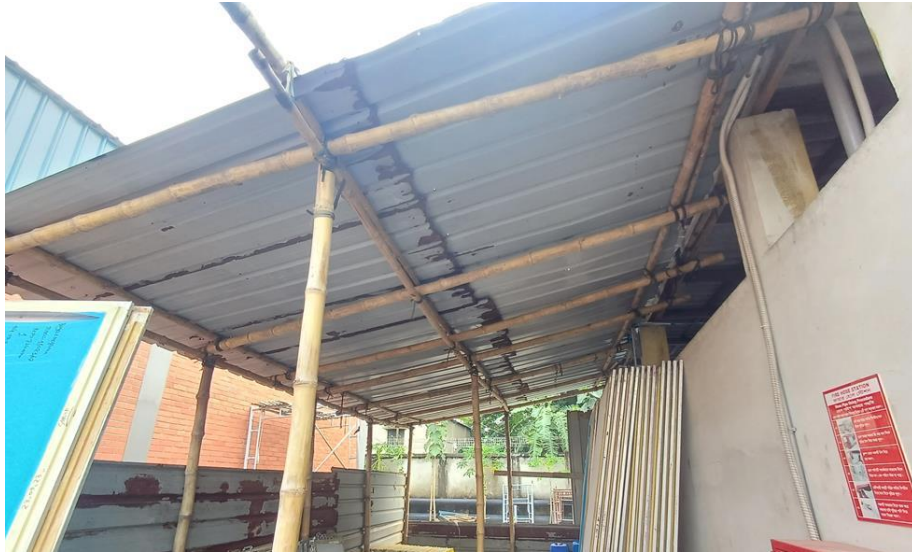
Apparently non-engineered structure with inadequate member and connection
