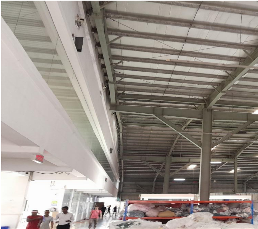
Mezzanine floor having no load plan
