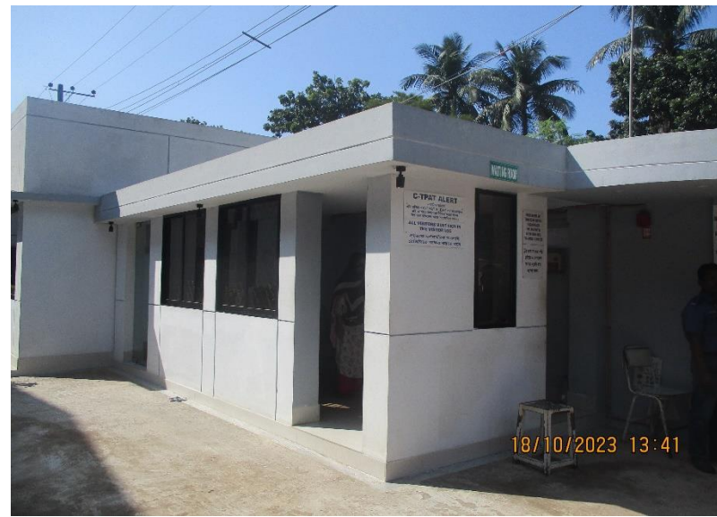
Fire command room
