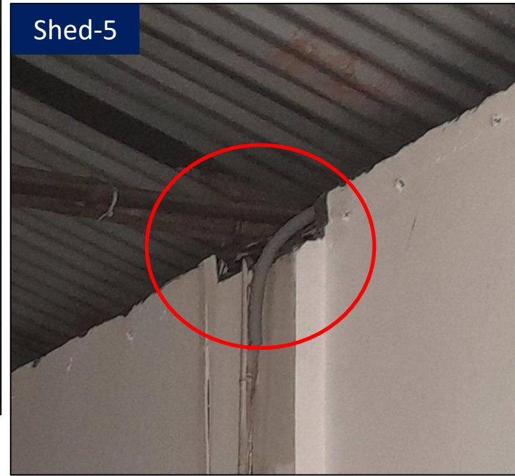
Truss welded with rebar of RC column
