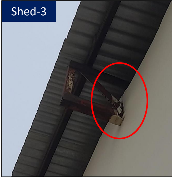
Purlin inserted to brick wall
