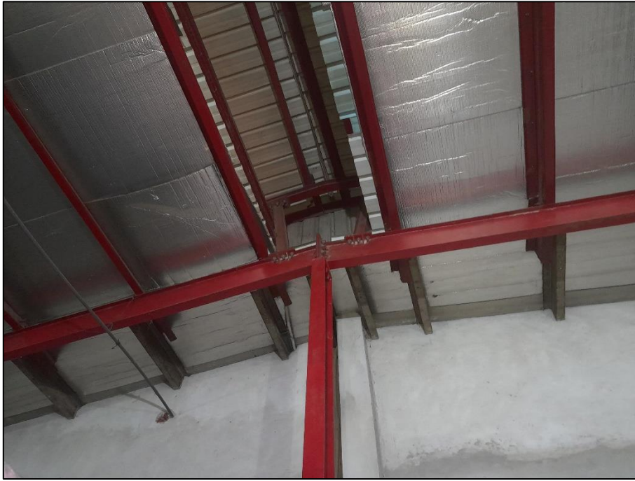
Portal frame along short direction.
