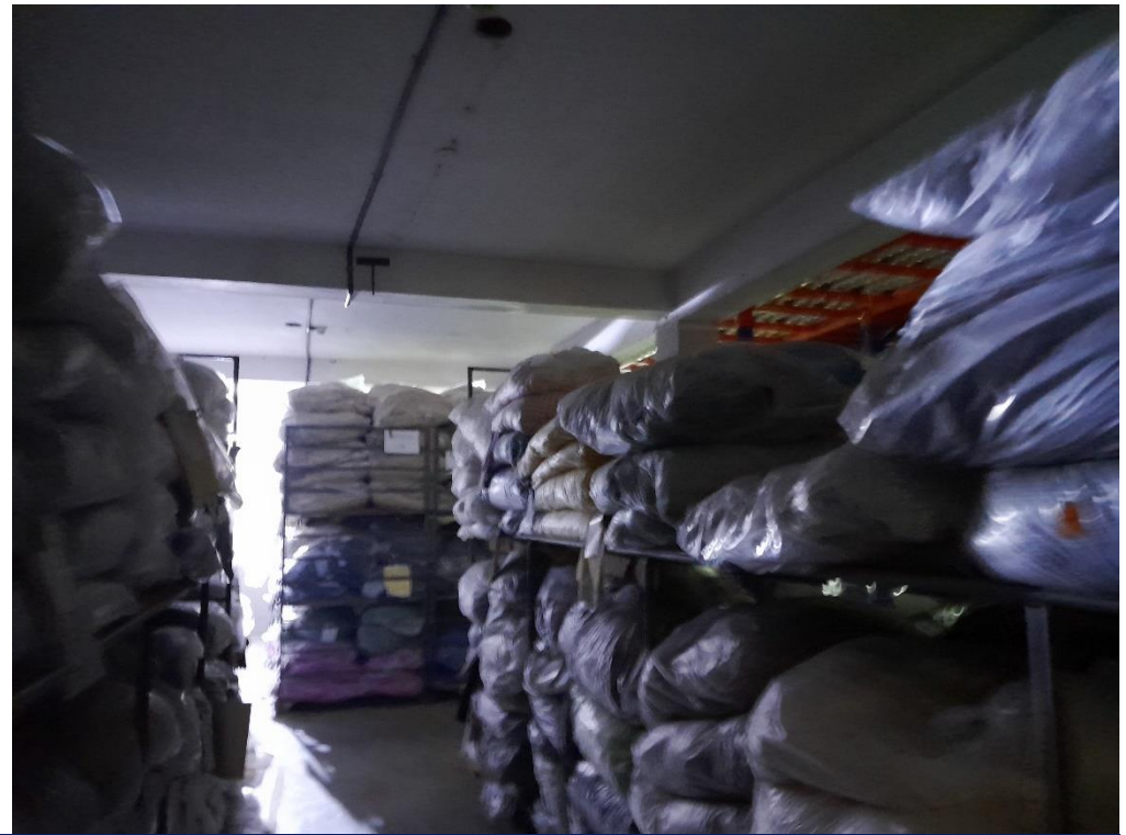
RC mezzanine structure.
