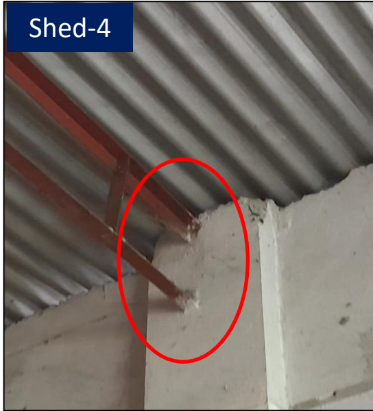
Purlin inserted to brick wall
