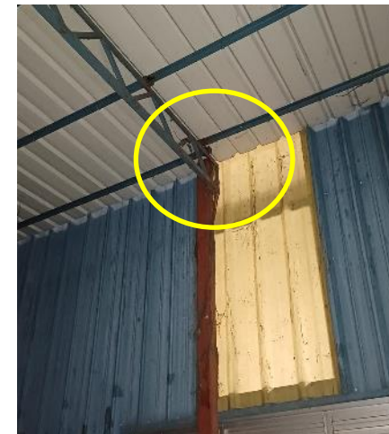
Apparently inadequate connection in store room
