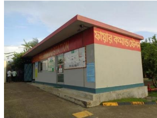
Security Post & Central Command Station
