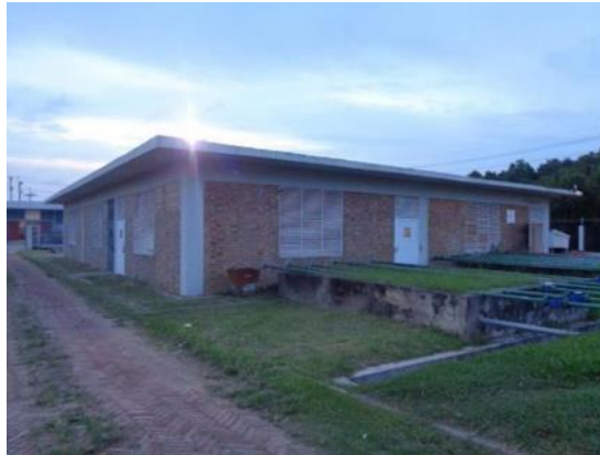
7 th phase Pump Room
