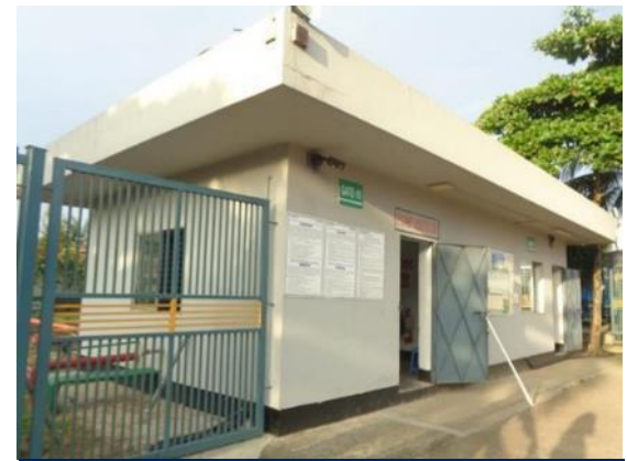
4 th phase Pump Room
