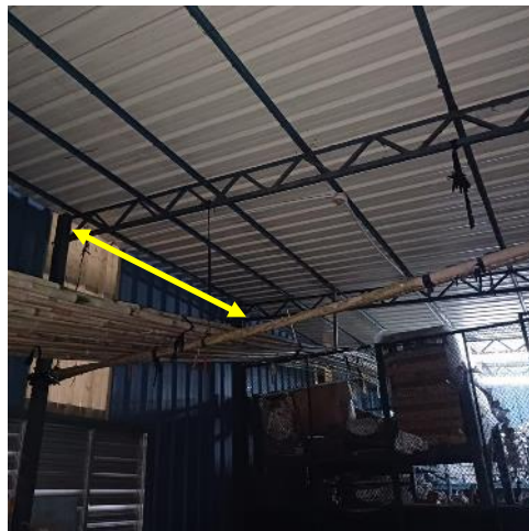
Lack of lateral stability in Temporary Garbage Store
