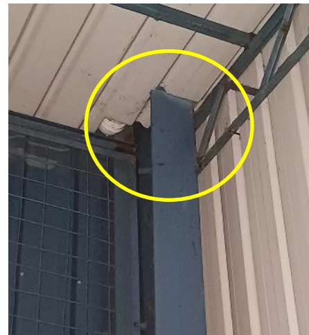
Apparently inadequate connection in store room
