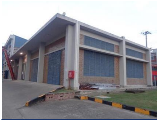
7 th phase sub-station
