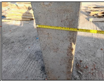
Column size measurement for C7 Column
