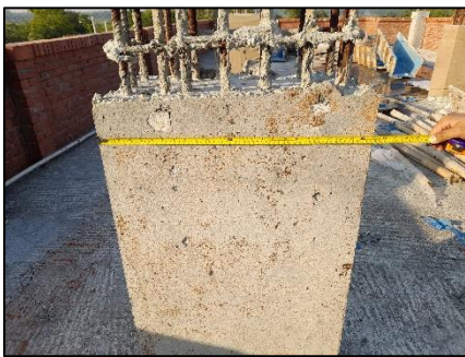
Column size measurement for C7 Column
