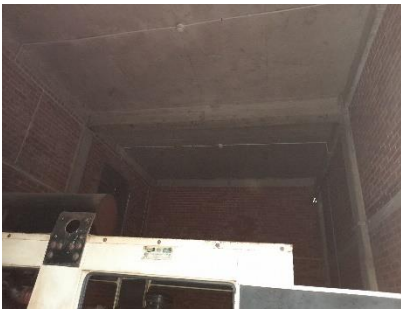
Interior of the utility building
