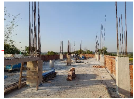
Re-bar number confirmed at roof
