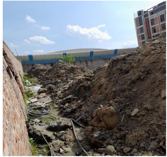
Earthwork ongoing opposite of the wall
