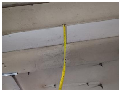
Ground floor onsite beam condition
