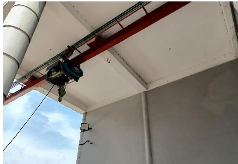
Overhang crane suspended from beam
