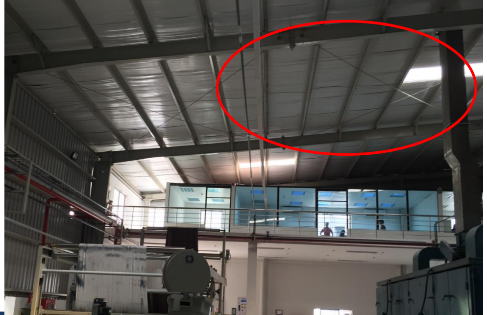
Cable bracing sagging in Production & Dyeing shed
