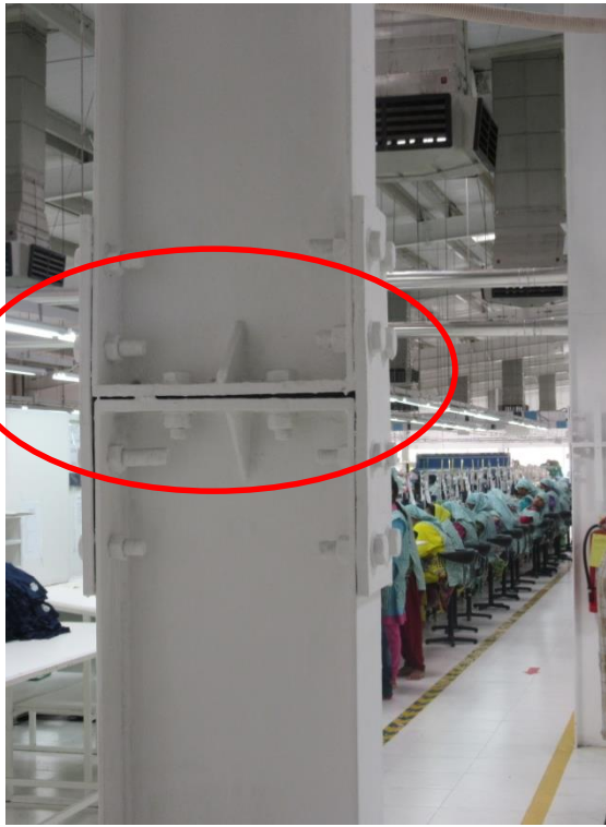
Poor connection in Production and Dining shed almost every column
