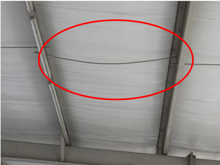
Cable bracing sagging in Production & Dyeing shed
