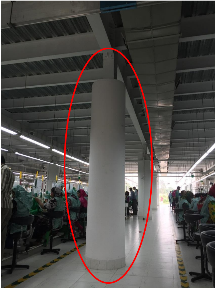
Steel posts supported on the RC columns from original design
