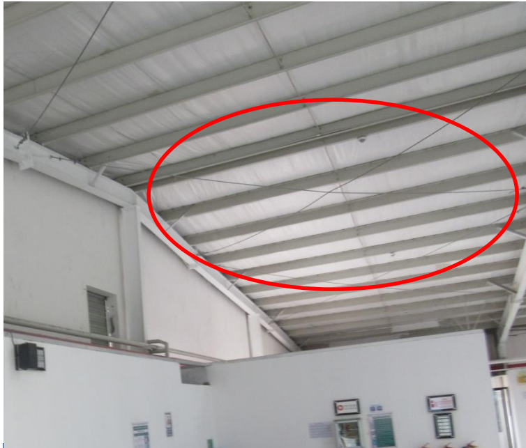
Cable bracing sagging in Production & Dyeing shed
