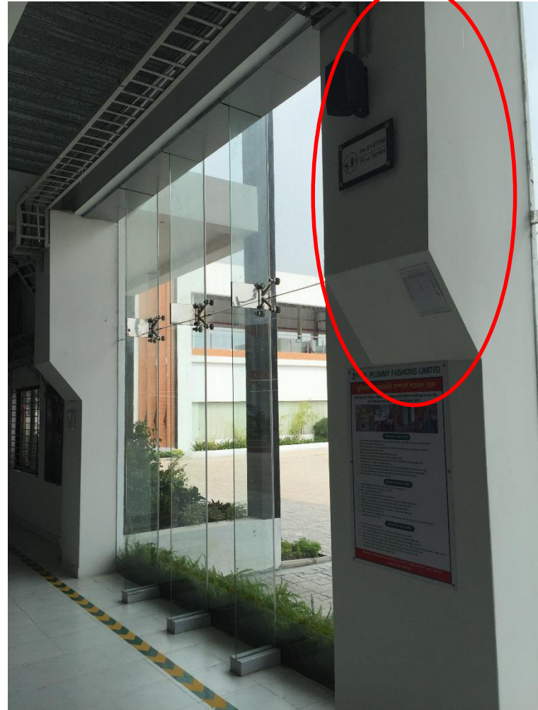
RC columns with corbels to support steel structure
