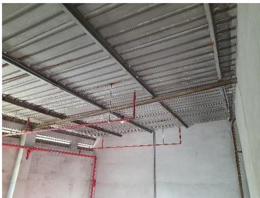
Steel Roof shed over the Fire pump room and control room
