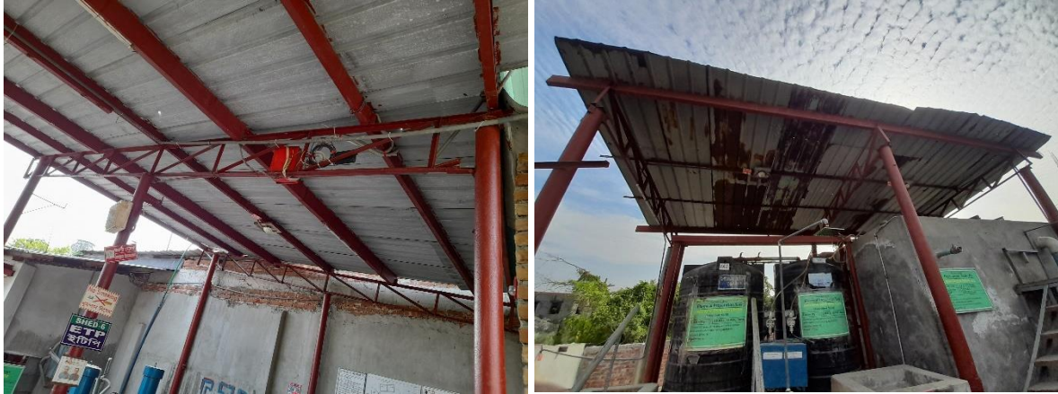
ETP steel shed
