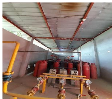
Missing edge beams at on-site condition
