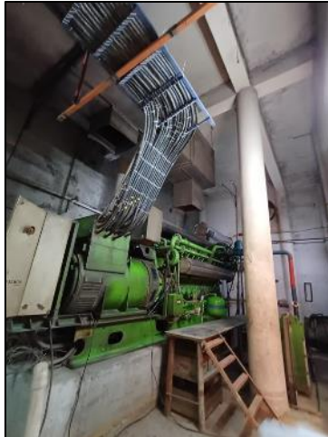
Building-9 (Generator Building)
