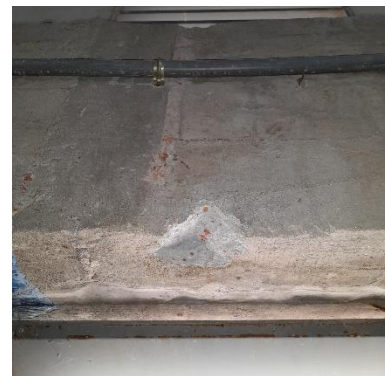
Beam aggregate-Brick chips
