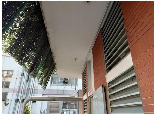
Cantilever slab
