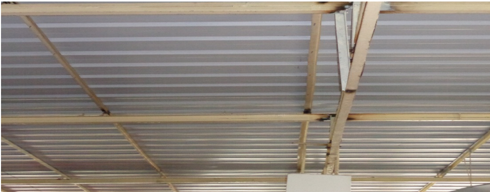
Roof at the garments building
