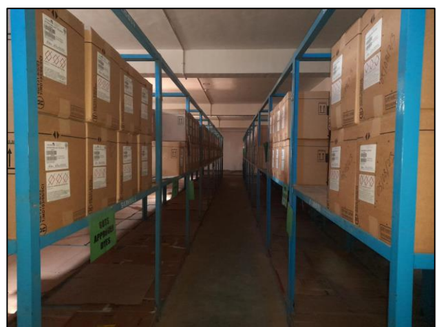
Unbraced storage racks on floors
