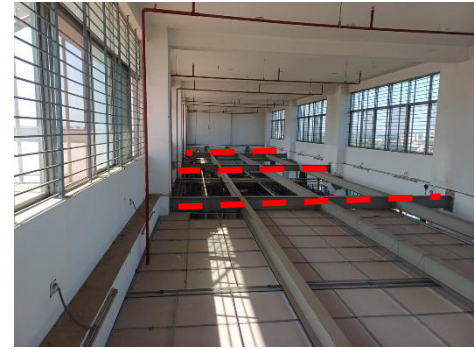
Steel beams instead of RCC beam were found at marked location of roof level (Block A).
