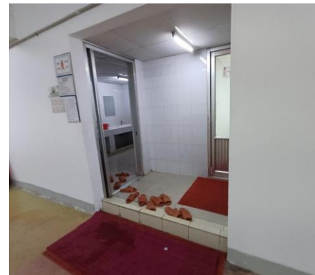
150 mm buildup at toilet area not mentioned in drawing.
