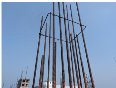
Exposed rebar at roof
