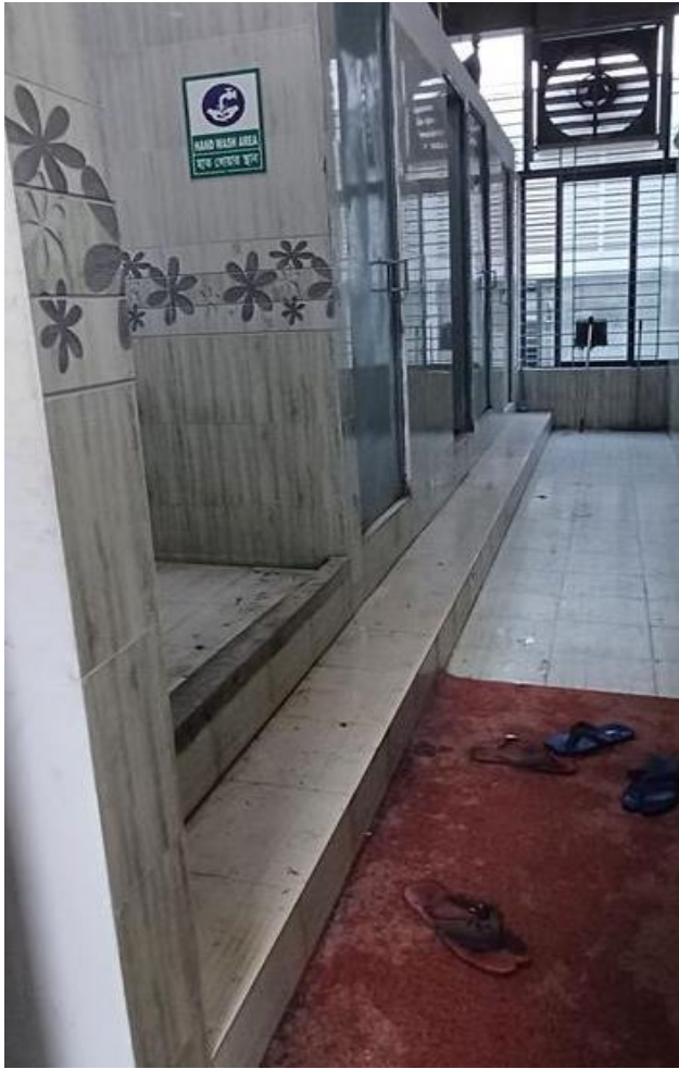
Floor build up found 450 mm
