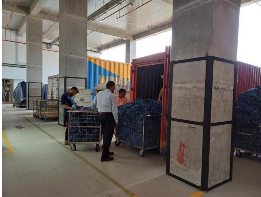
Barrier connected to column directly
