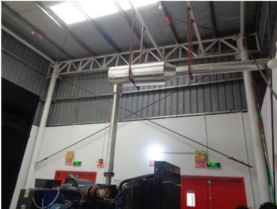
Vertical bracing at half-length of pipe column.
