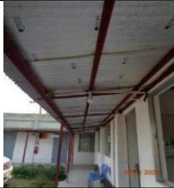
Lightweight steel roof supported by periphery brick wall
