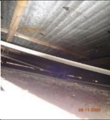
Bamboo rafter with tin roof supported by brick wall
