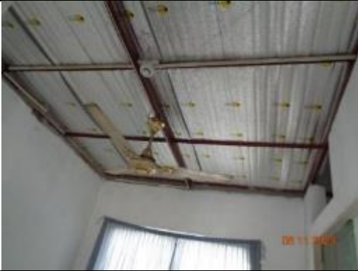
Lightweight steel roof supported by periphery brick wall
