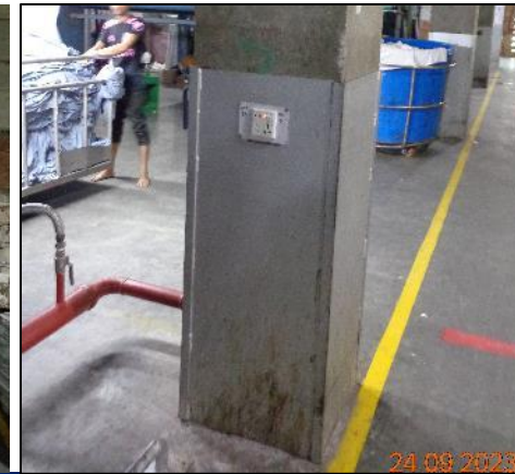
Electric duct in RC Column at Ground floor
