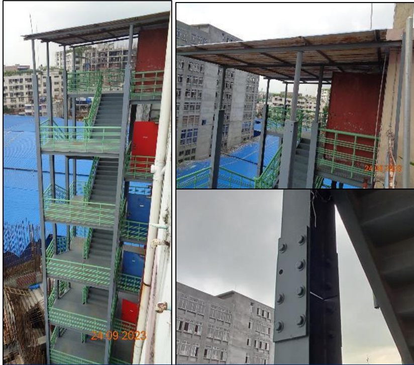
Light weight non-engineered roof shed over the steel stair-1.
