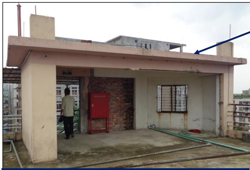
Stair top beam column framing
