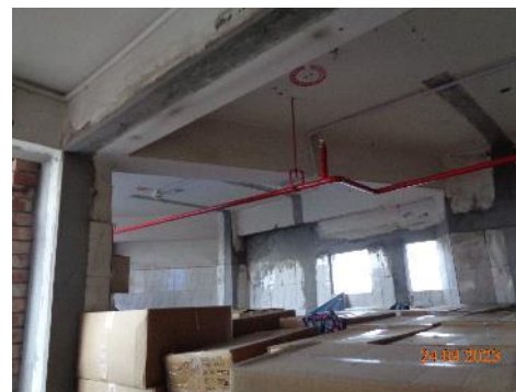
Beam layout mismatch
