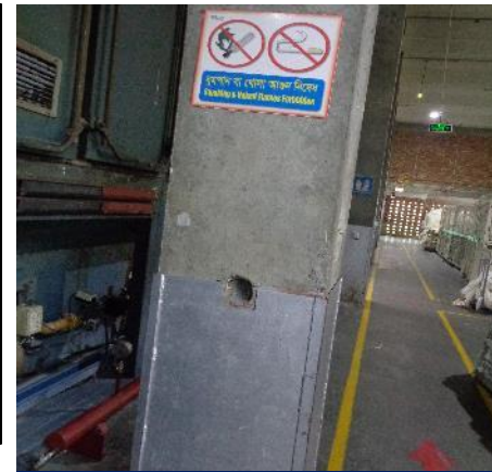
Electric duct in RC Column at Ground floor
