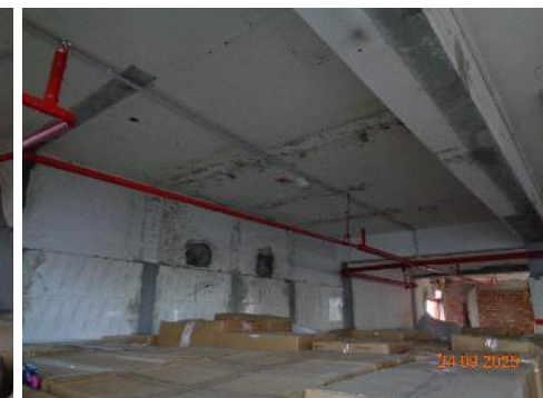
Beam not found at site
