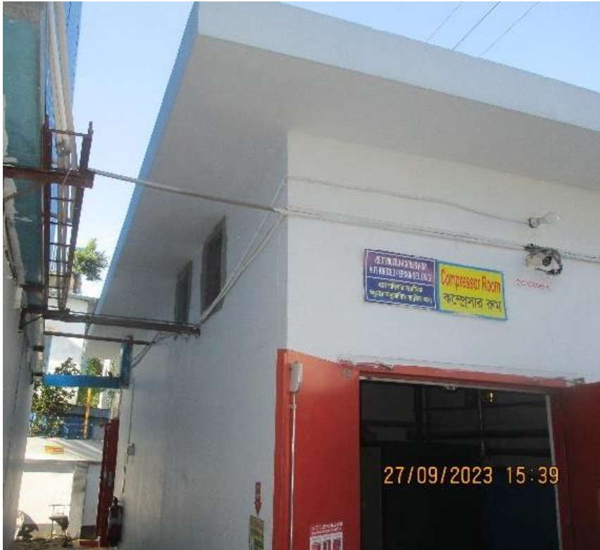
Compressor & Boiler Room
