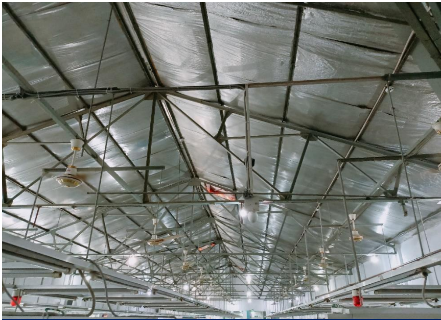
Typical truss frame without bracing
