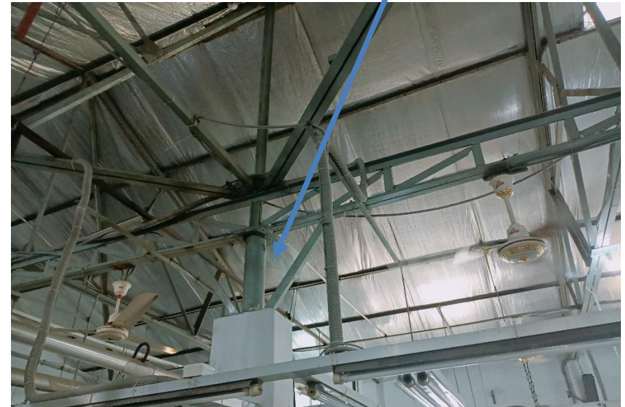
Truss junction on steel column
