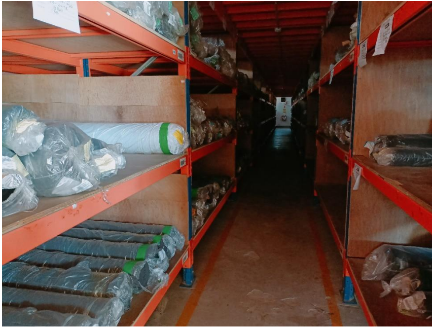
Non-anchored storage rack at several floors
