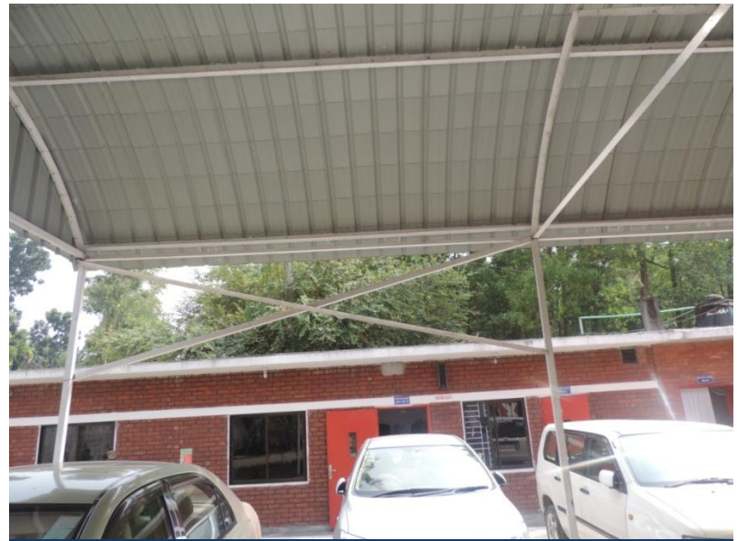
Non engineered structure
