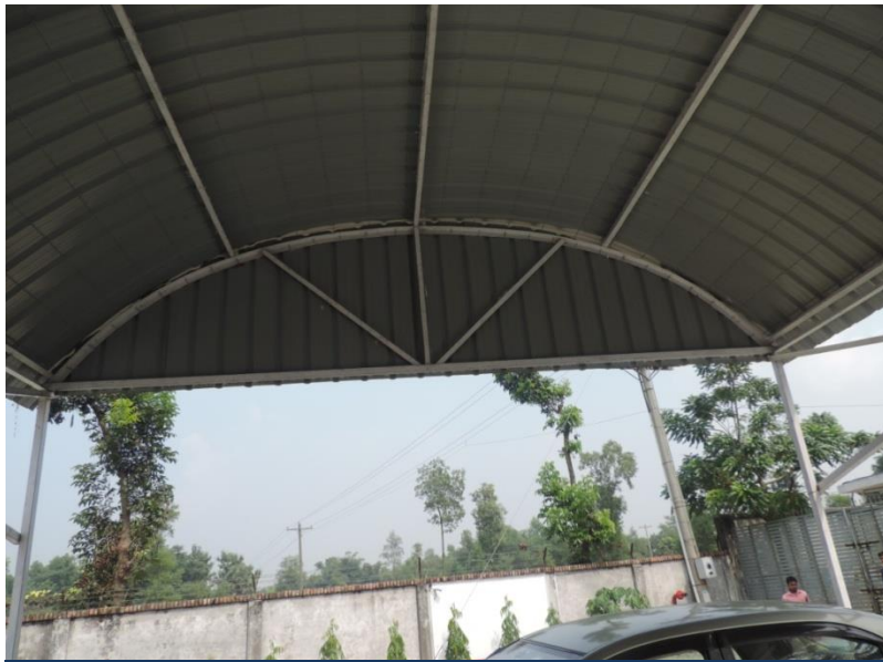
Non engineered structure
