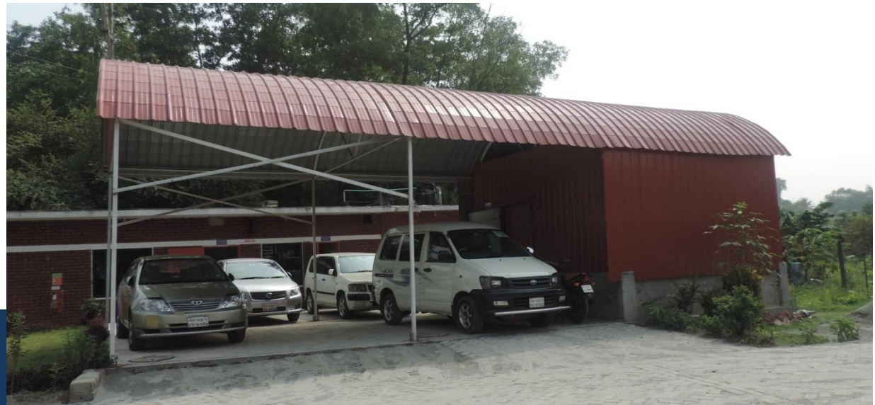
Structure is open to impact by cars
