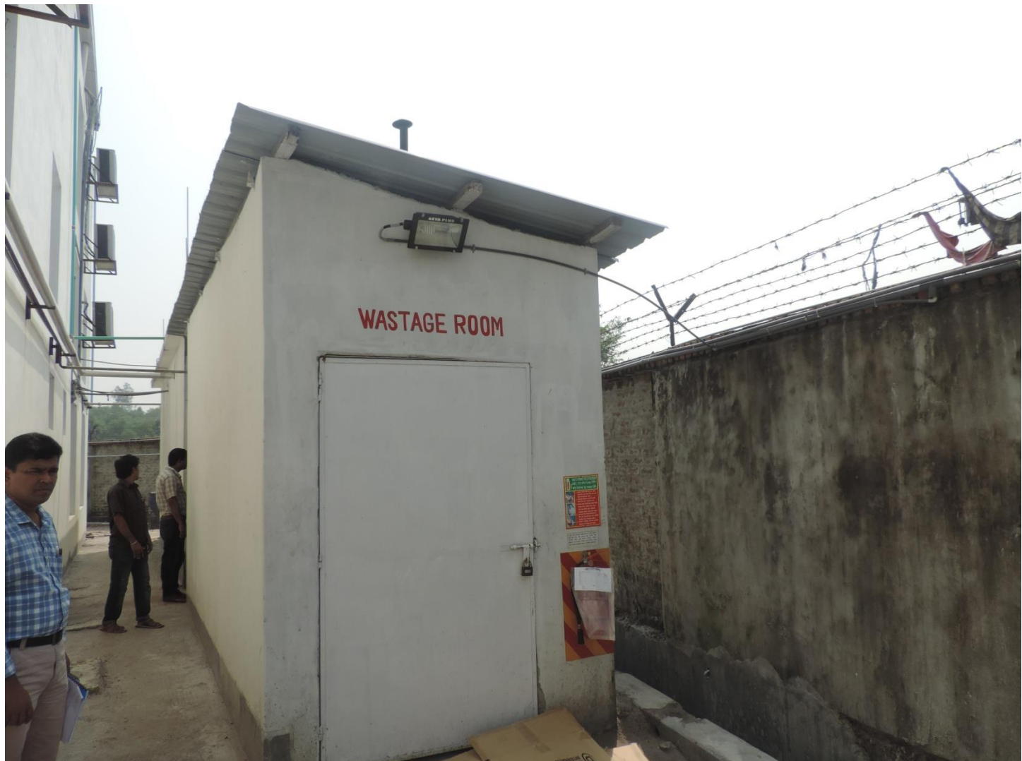
Non engineered roof
