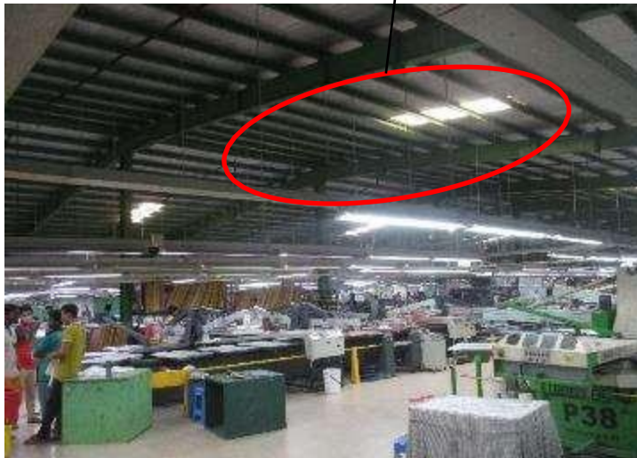
No horizontal pipe bracing was observed
