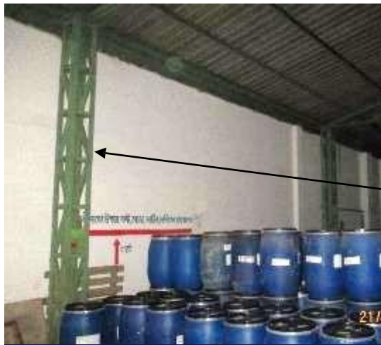
Truss is supported by steel lacing column
