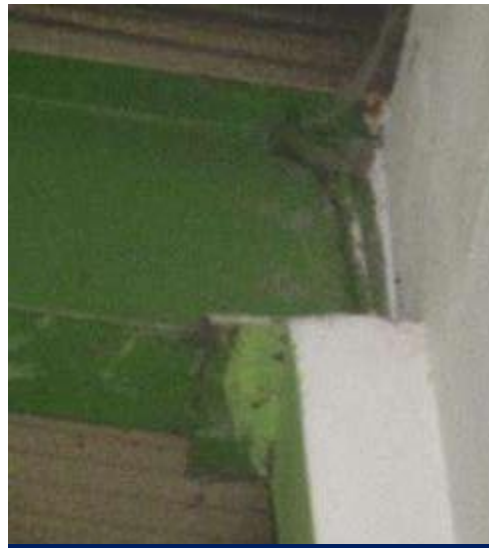
RC column and rafter joint on edge
