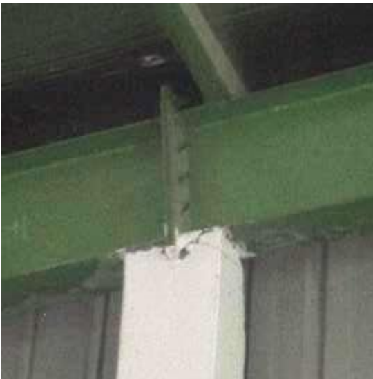
RC column and rafter joint on end bay
