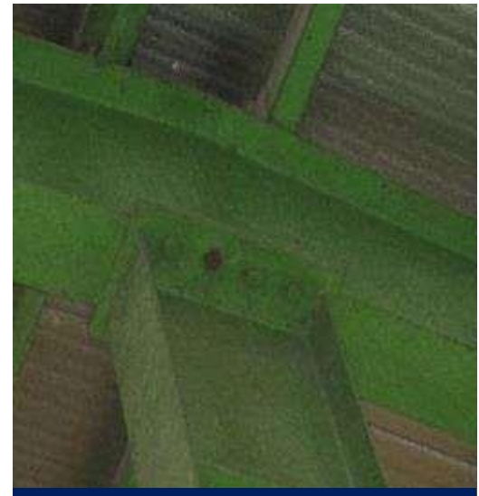
Steel column rafter joint at middle
