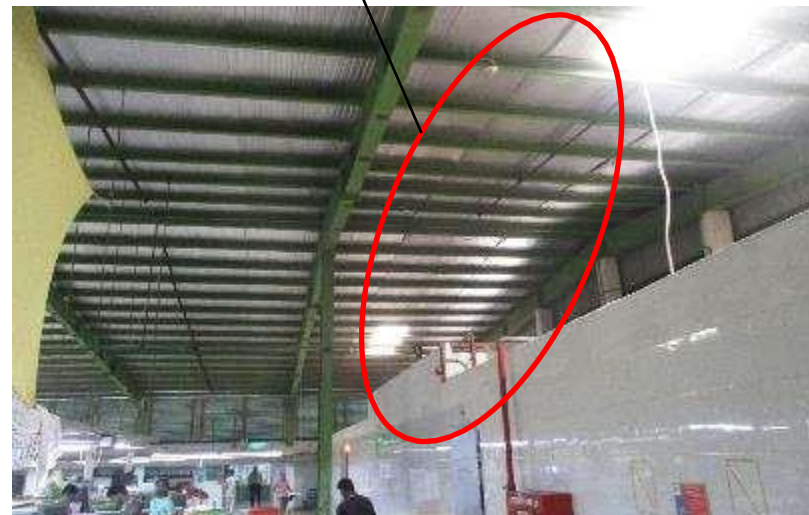
No horizontal pipe bracing was observed
