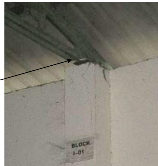
Edge of truss is supported by RCC column
