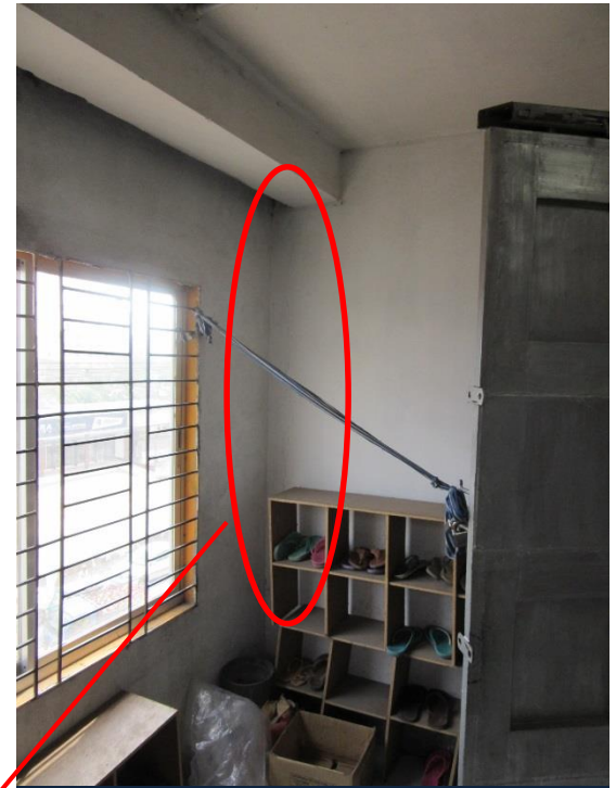
North staircase. 1st Floor
