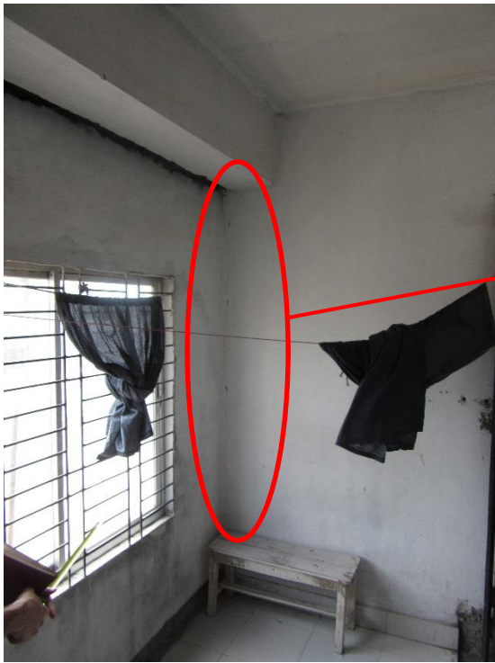
North staircase. 2nd Floor
