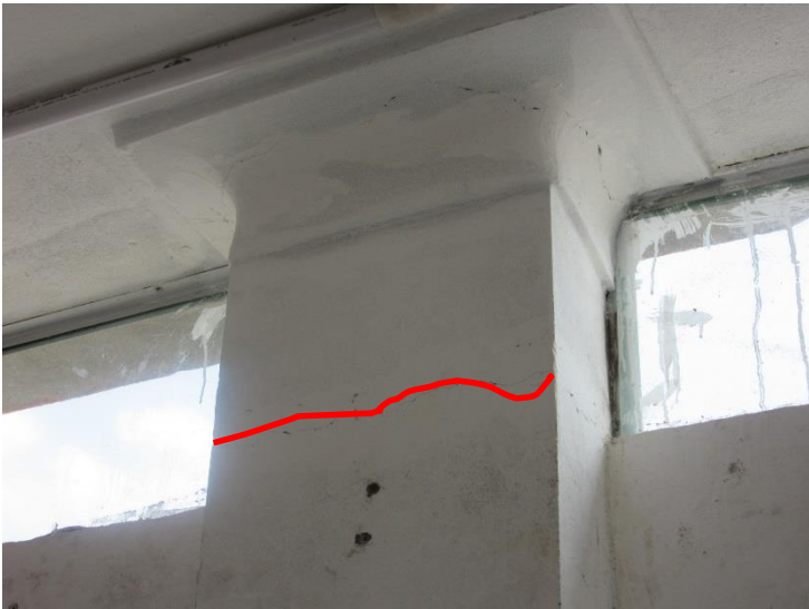
West Facade pillar
