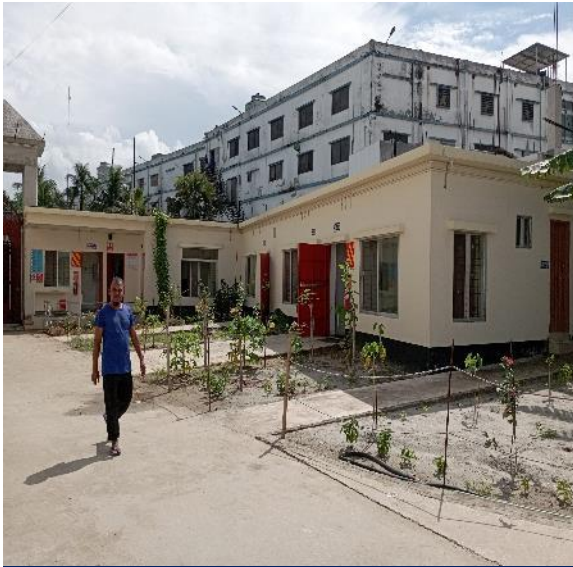
Medical, Daycare & Security Room
