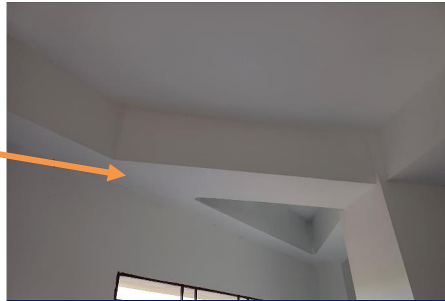
Beam layout does not match with drawing
