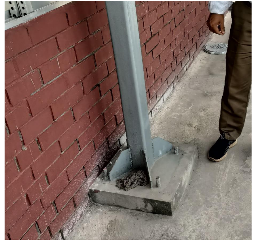
Nut missing in several bolts
