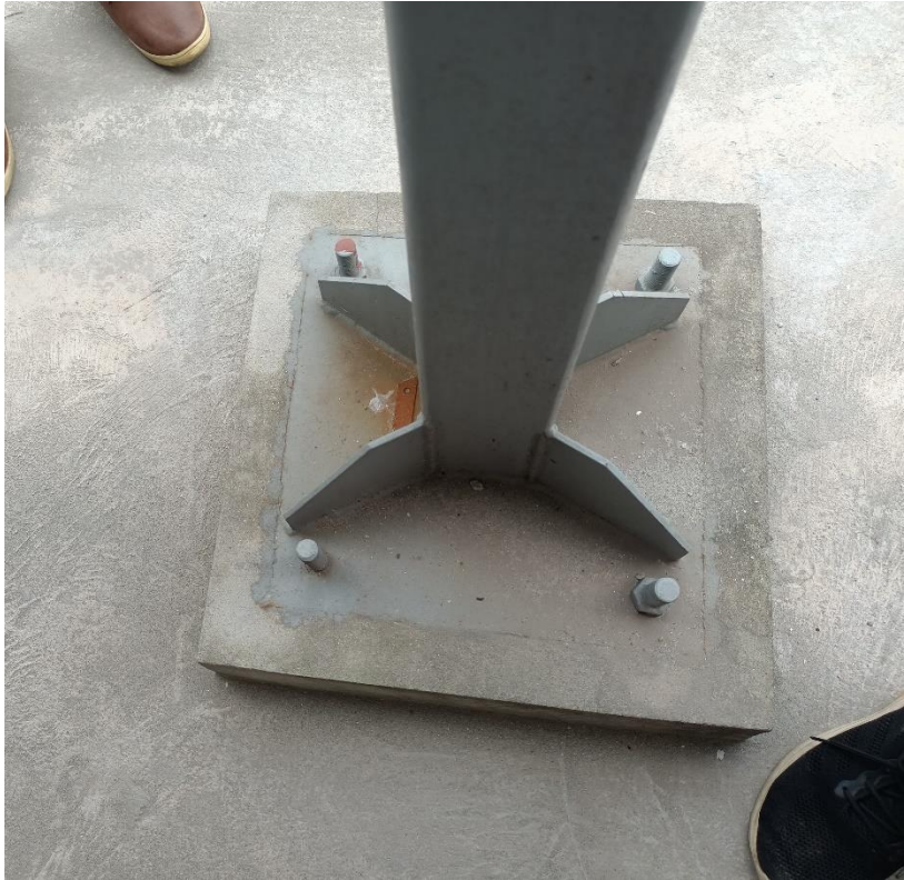
Nut missing in several bolts
