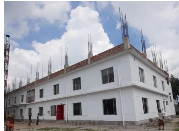
Building constructed up-to two storied. Extended column re-bar at roof/2 nd floor
