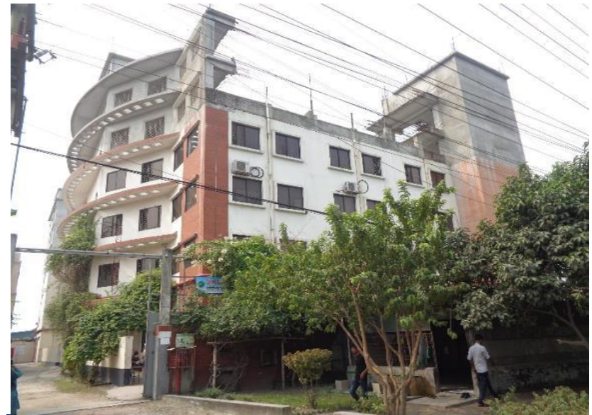
Building is currently 4 storied
