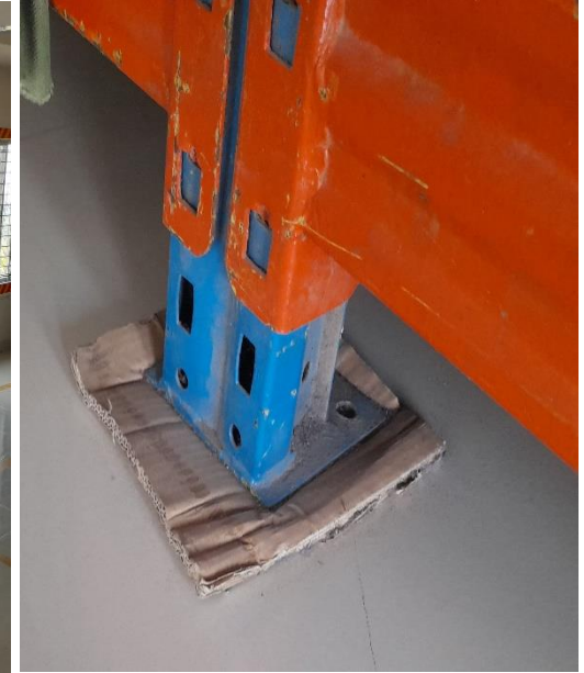
Storage rack found within the building without braced/anchored
