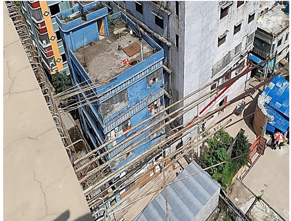
Exposed reinforcement left at each level
