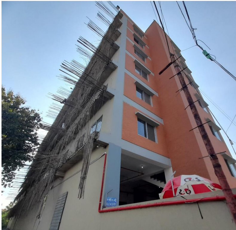
Exposed reinforcement left at each level
