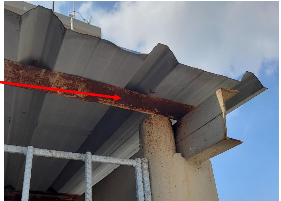
Corrosion on steel member
