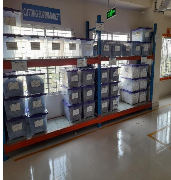
Storage rack found within the building without braced/anchored
