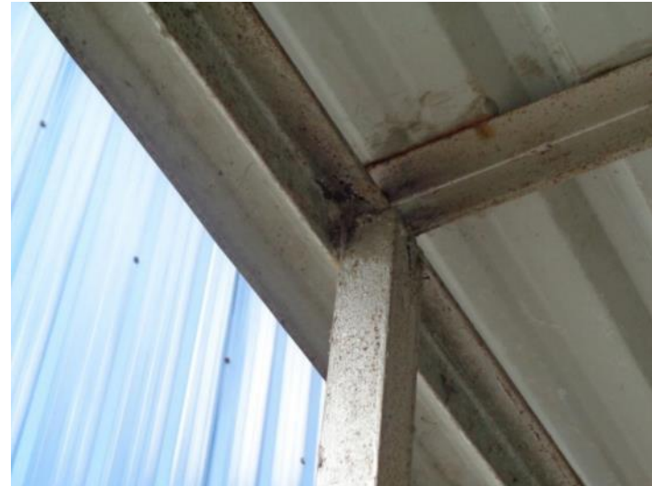
rafter and steel column connection
