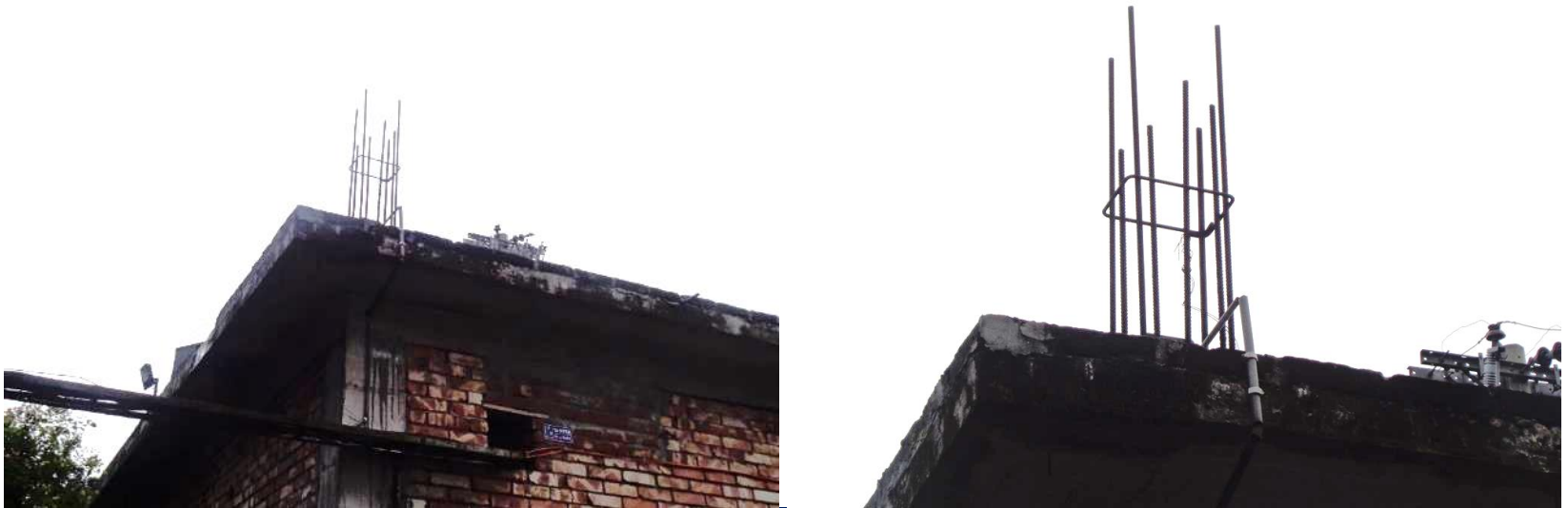
Exposed rebar on roof
