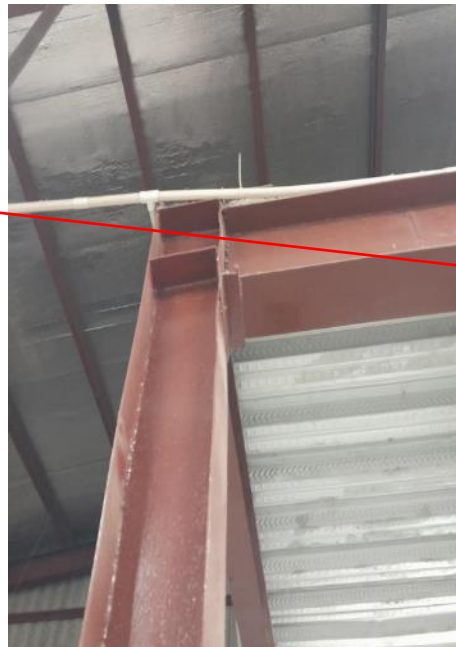
Distorted steel beam-column joint
