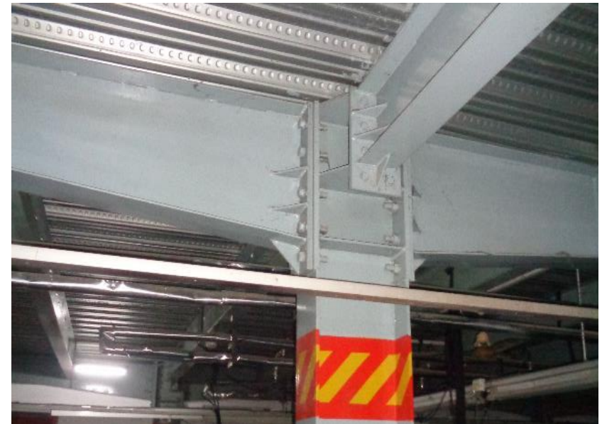
Connection of Main Beam to Column
