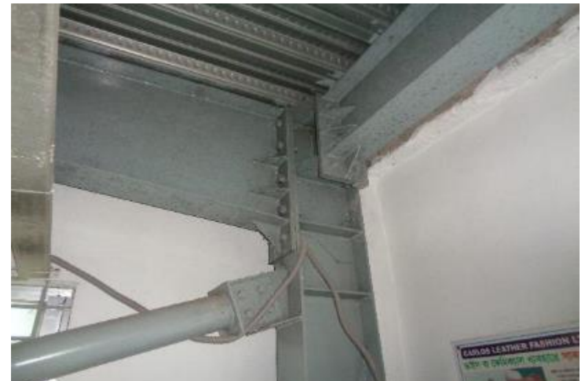
Connection of Bracing to Column
