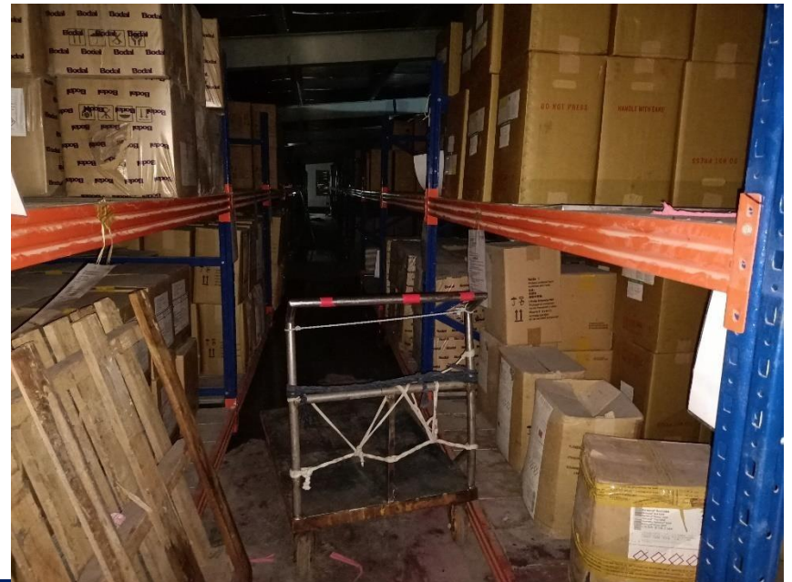
Non-anchored storage rack at first floors
