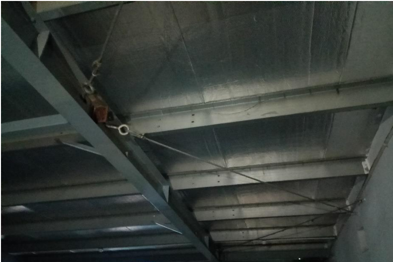
Missing compression strut member
