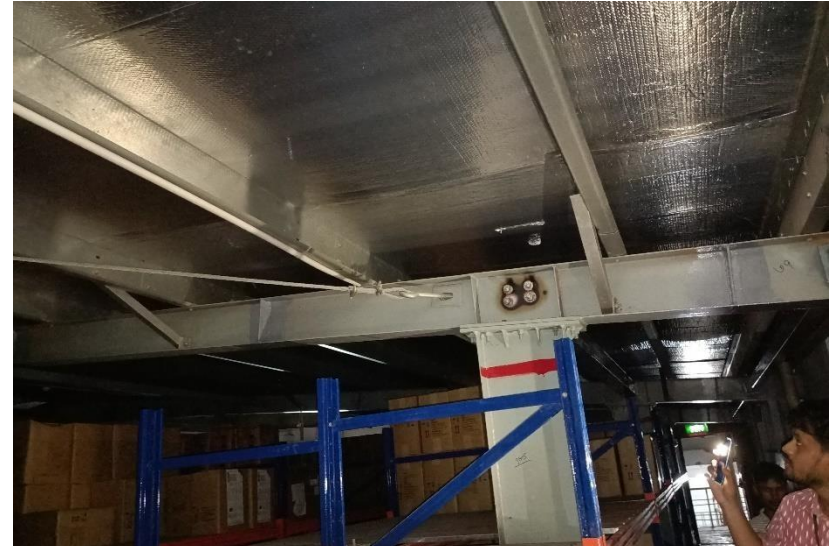
Missing compression strut member
