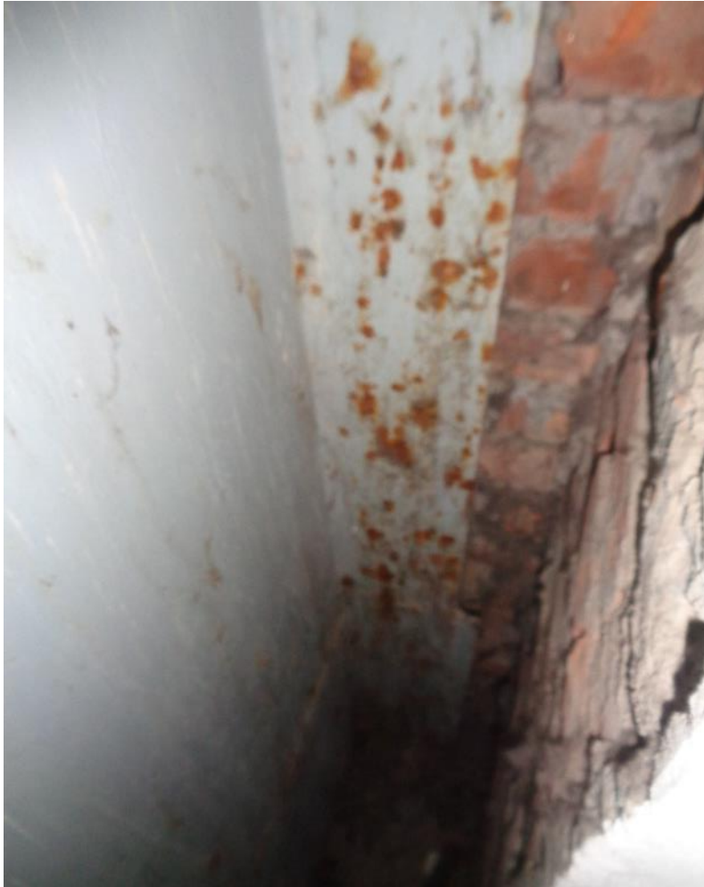
Corrosion in steel column
