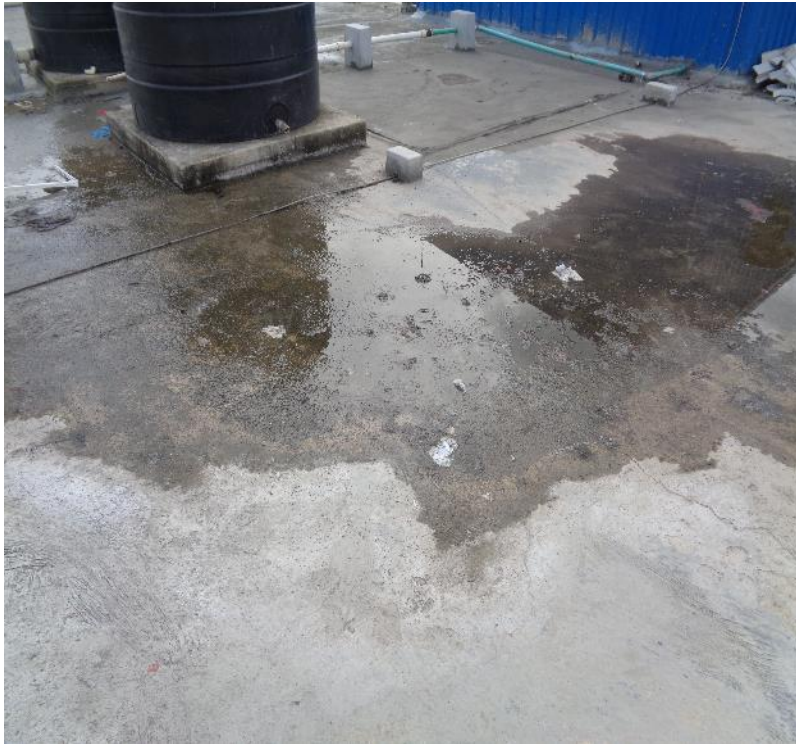
Water ponding on roof slab due to poor drainage system
