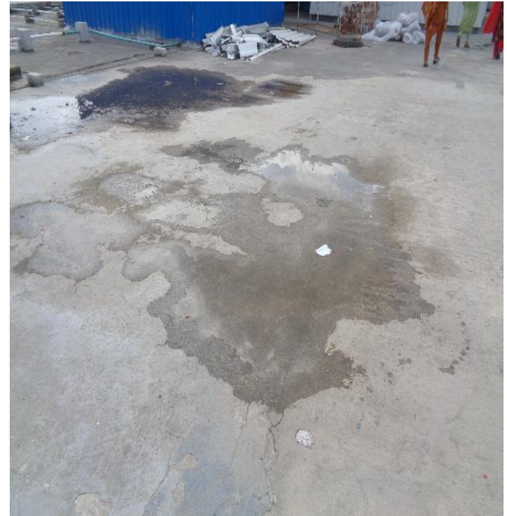
Water ponding on roof slab due to poor drainage system
