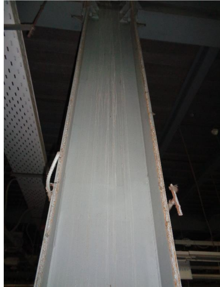
Corrosion in steel column
