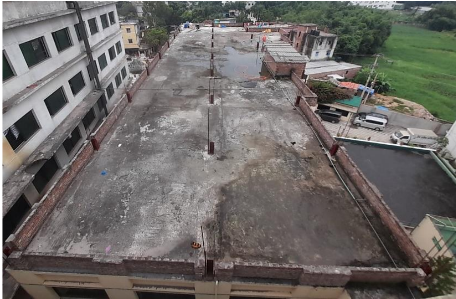
Water ponding on roof slab due to poor drainage system
