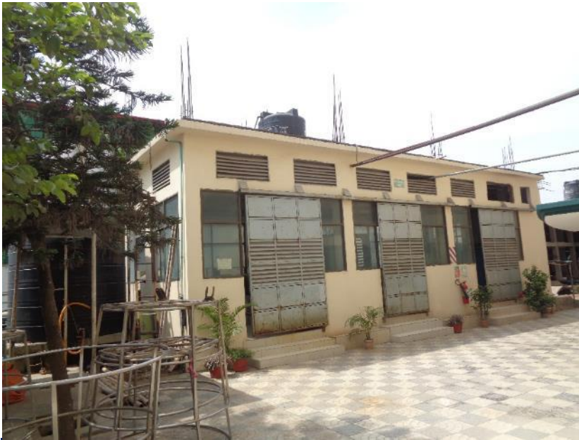
ETP Control Room
