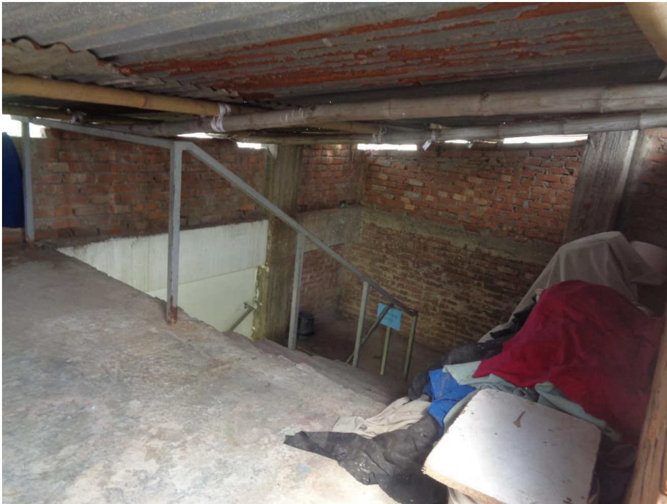
Bamboo shed over staircase
