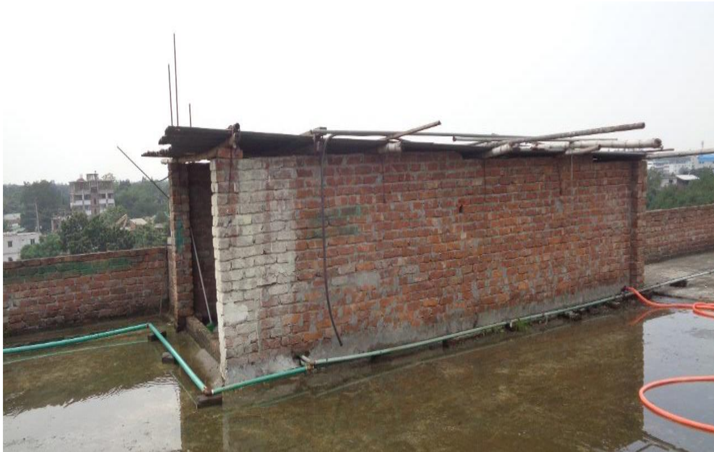
Non-engineered bamboo shed over staircase
