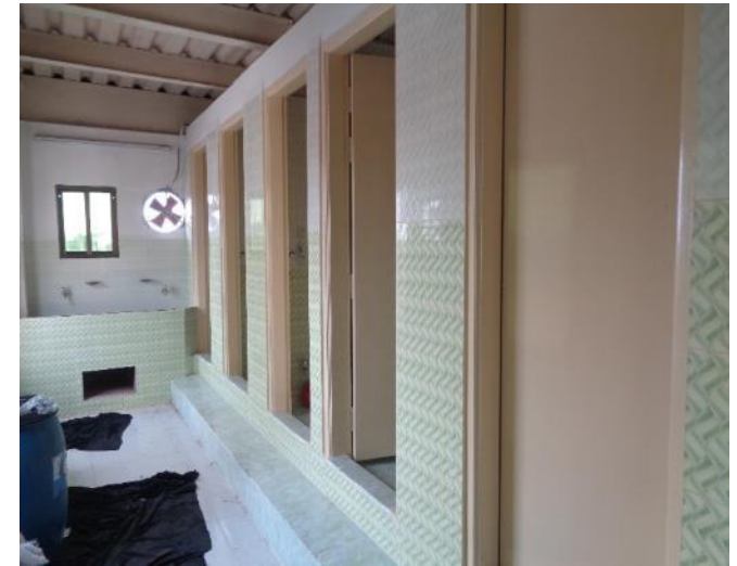
Source of loading: Toilet build up and partition wall on 2 nd floor
