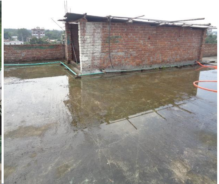
Water ponding on roof slab due to poor drainage system
