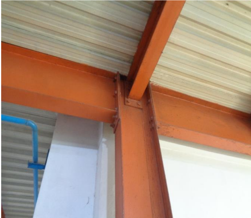
Moment frame in E-W direction
