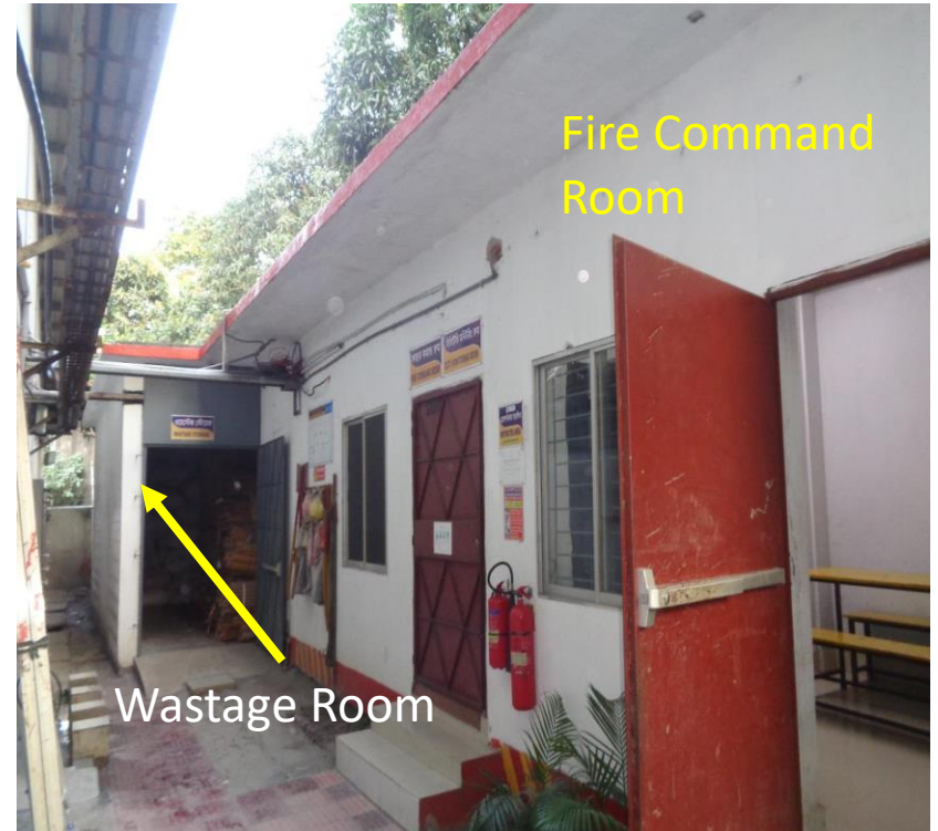
Wastage Room and Fire Command Room
