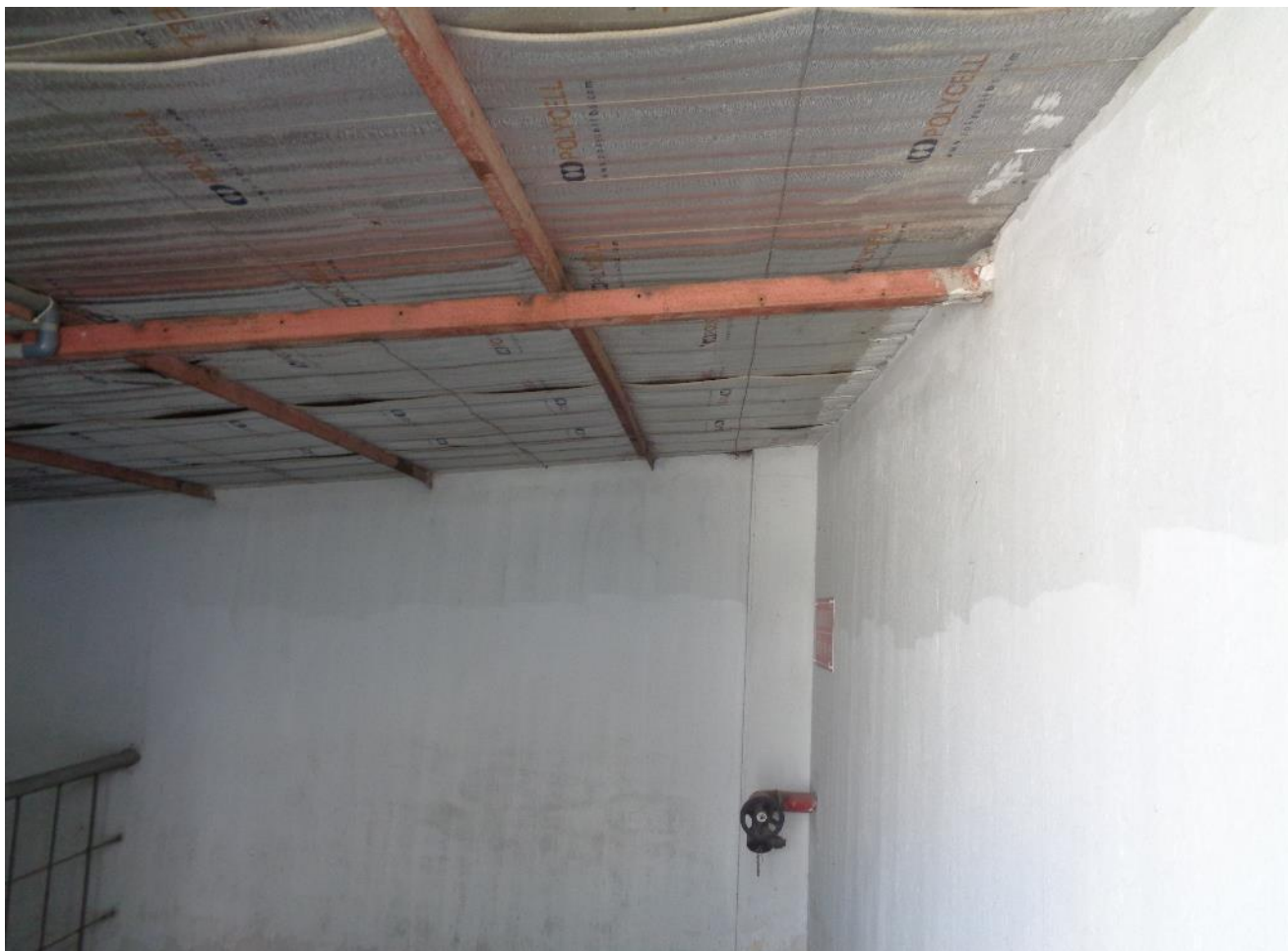
Steel members inserted to brick walls.
