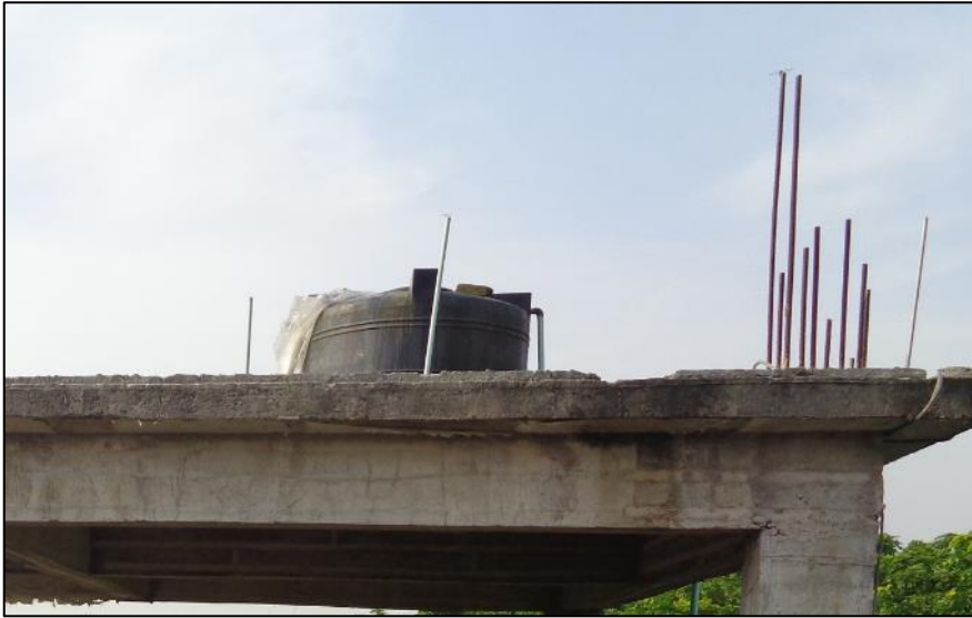
Exposed rebar at roof
