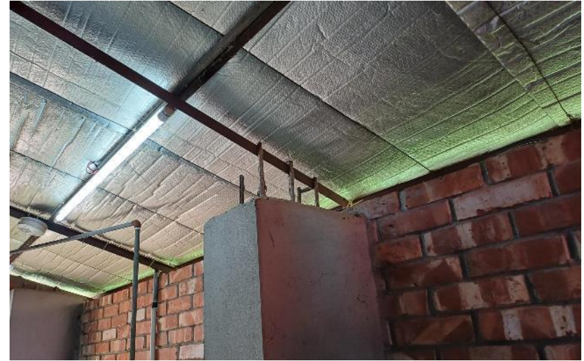
Lightweight roof shed
