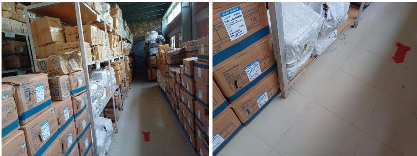
Steel racks without anchored/braced.
