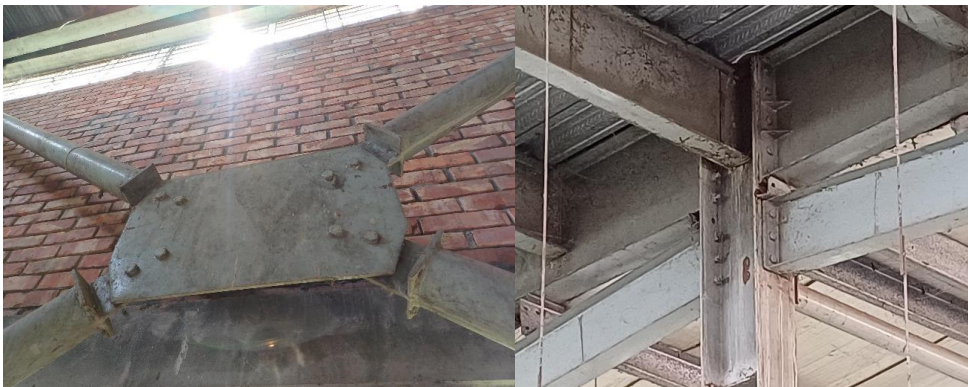
Bracing Connection and Column & Beam connection
