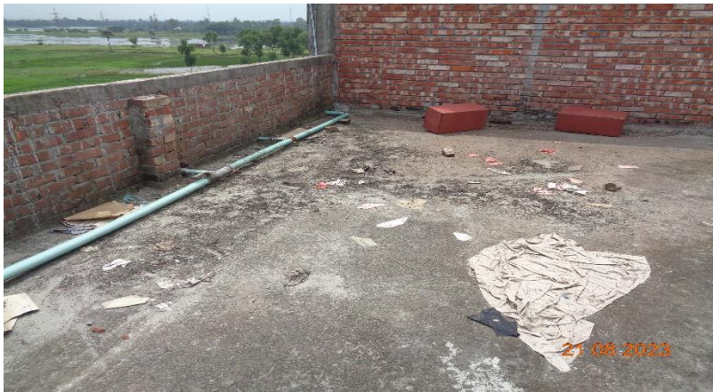
Water ponding signage at roof
