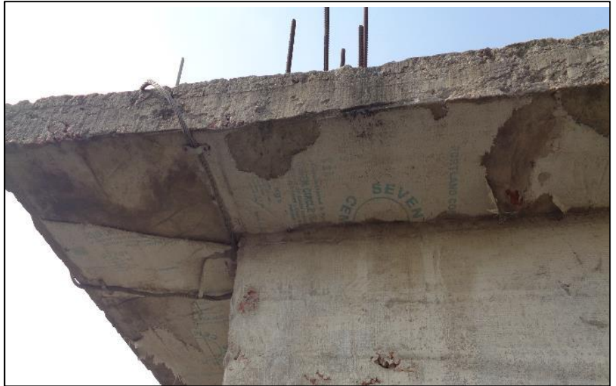
Exposed rebar at roof
