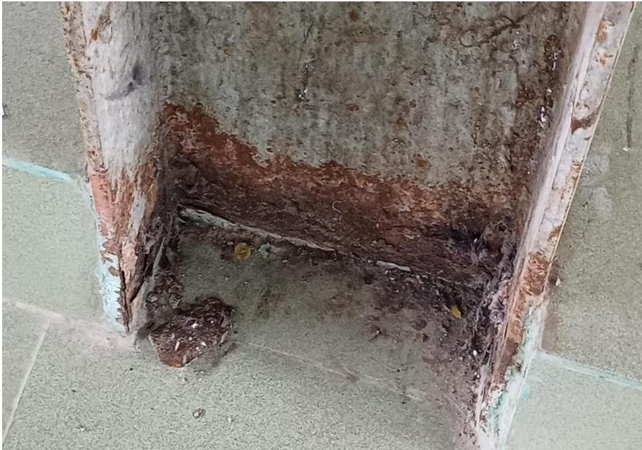
Corrosion in steel member
