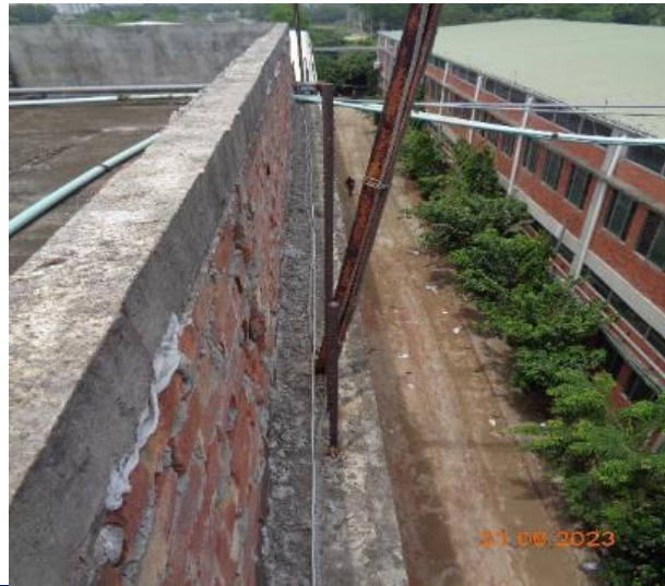
Exposed corroded rebar at roof
