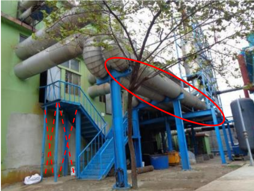
Lack of load transfer media along east-west dir.
