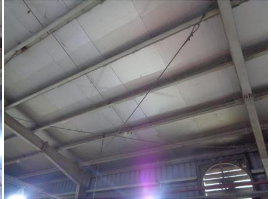
Loose cable bracing
