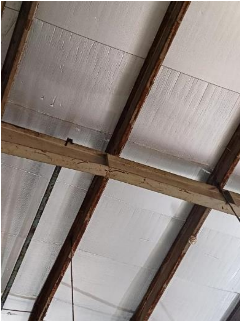
Several corroded steel members at the roof
