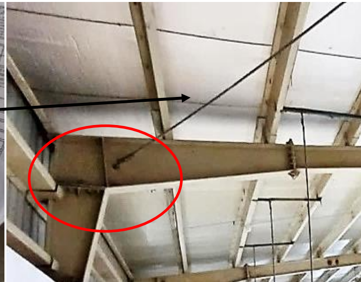
Bracings were connected apart from column-rafter joint
