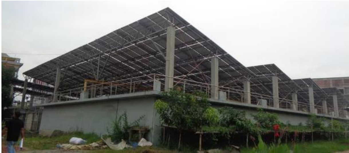
New ETP roof structure
