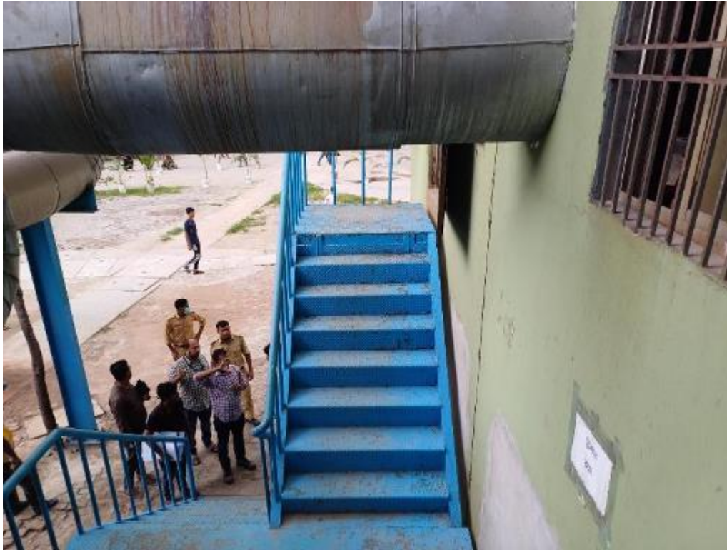
Corroded steel stair
