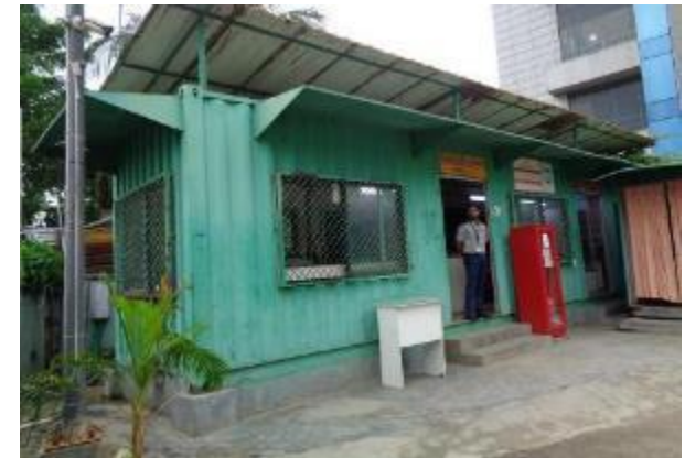
Lack ground anchorage and foundation system for ancillary 4, 5 & 6 (General Security Post, Female Security Post and Container Security Office at main gate)
