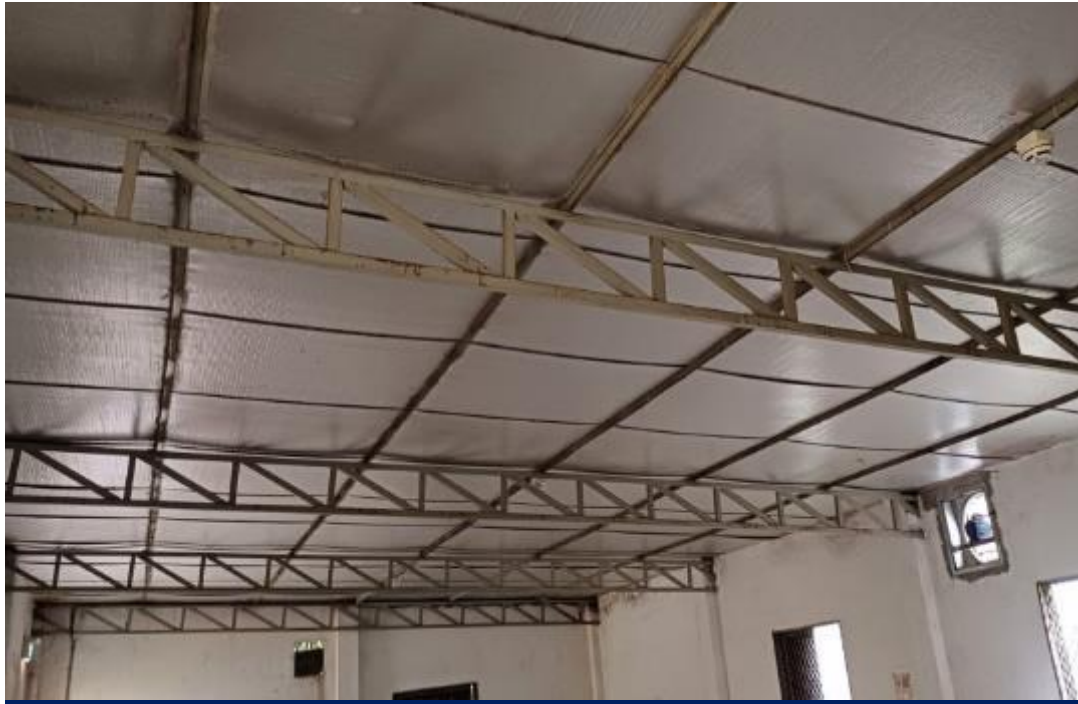
Roof truss connected to brick wall
