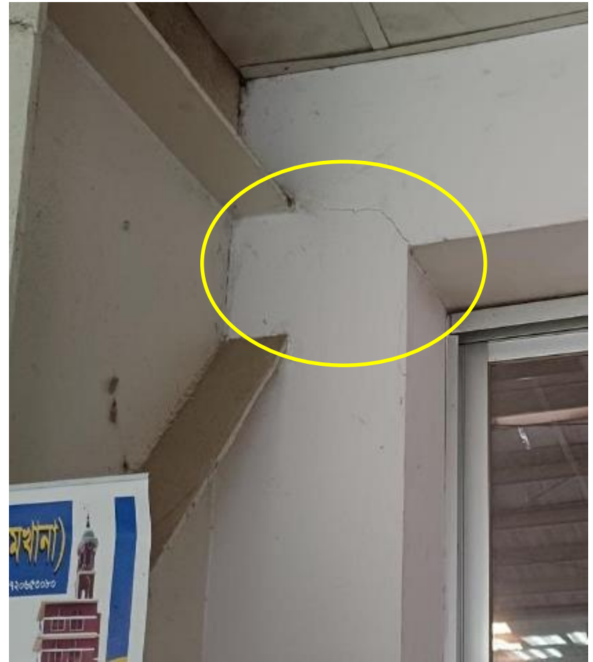
Crack on wall at several locations
