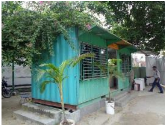
Lack ground anchorage and foundation system for ancillary 4, 5 & 6 (General Security Post, Female Security Post and Container Security Office at main gate)
