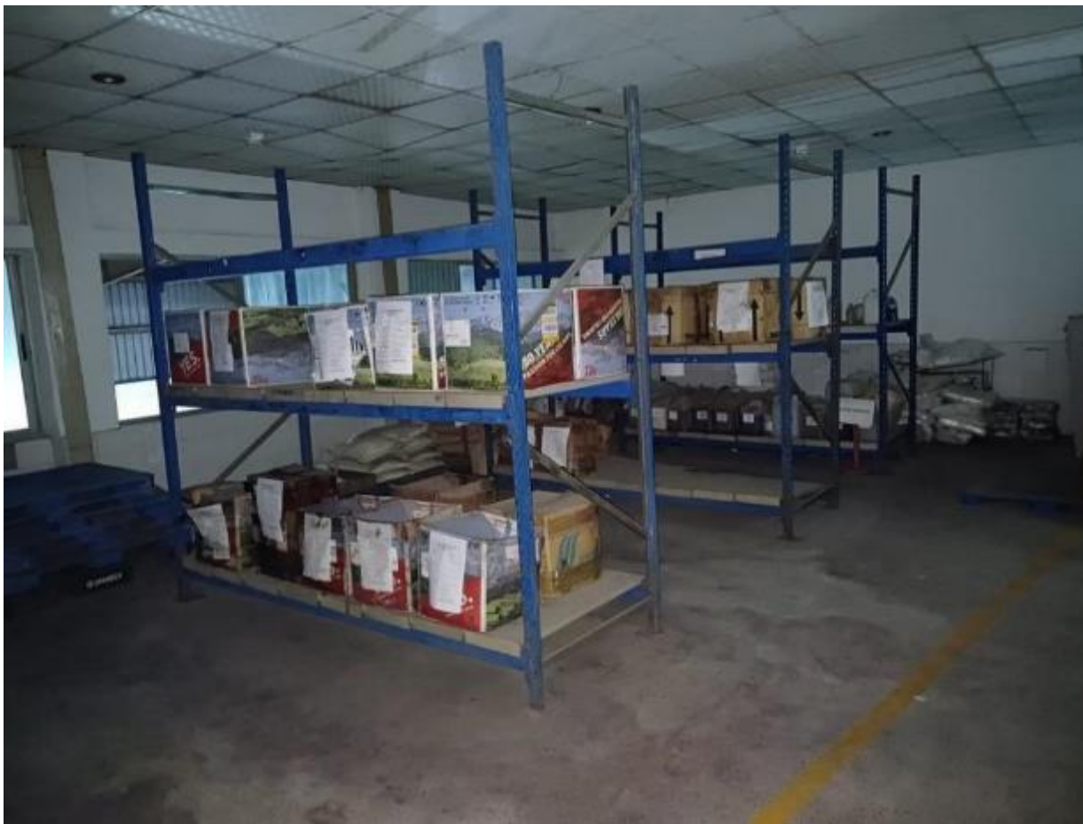
Storage rack found within the building without braced/anchored
