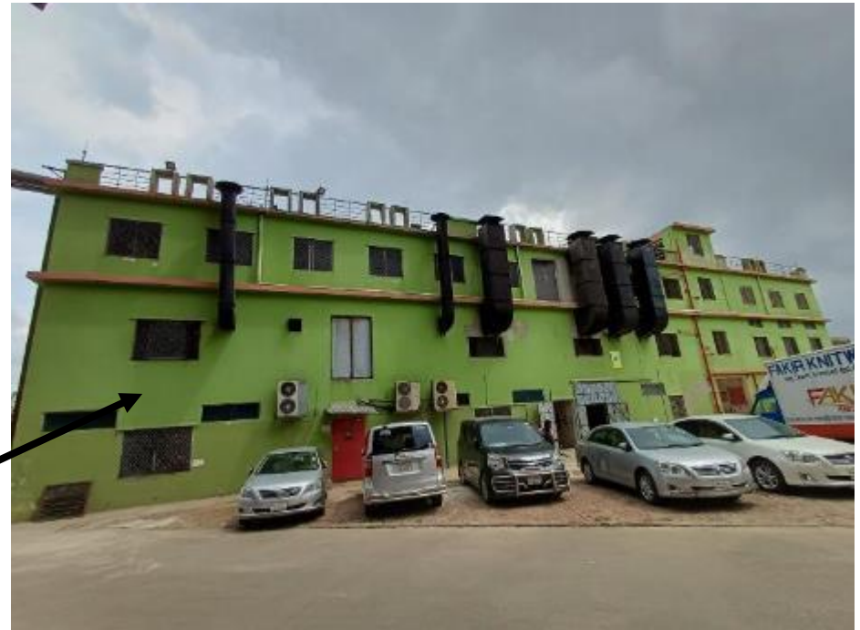
As-built construction of Building-4: 3 storey
