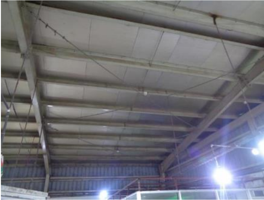
Loose cable bracing
