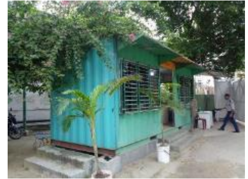
4. General Security Post, Main Gate
