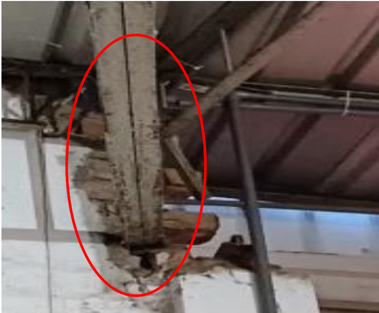
Truss is inserted to brick wall
