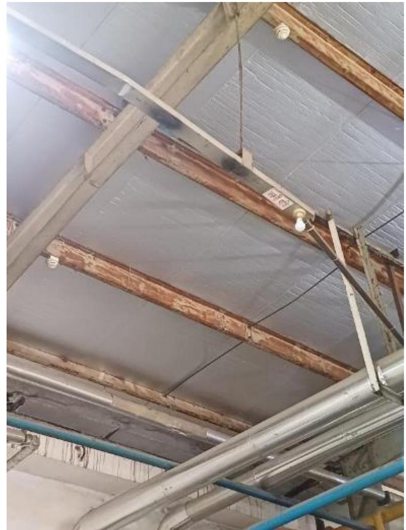
Several corroded steel members at the roof
