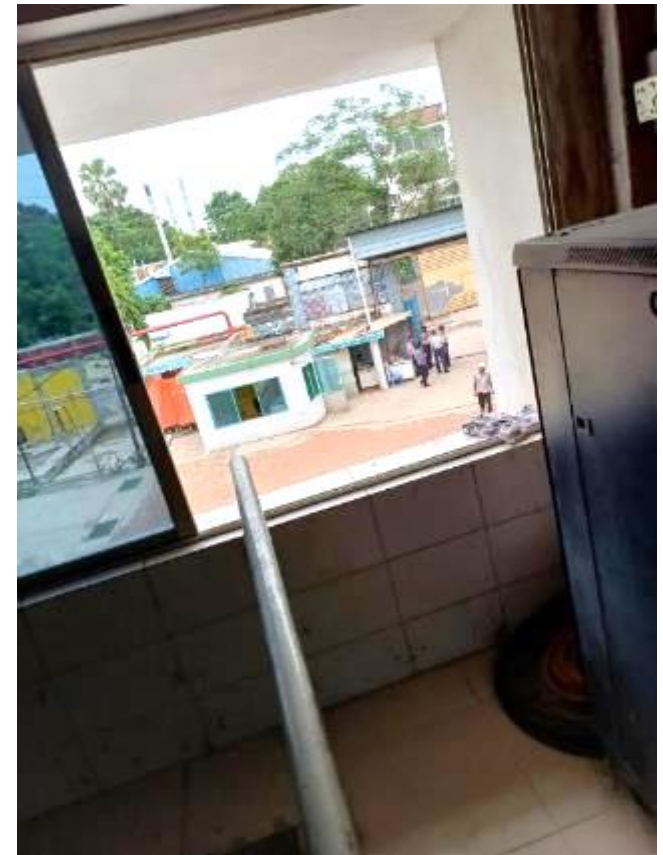
Falling hazard at mezzanine floor due to low height masonry wall
