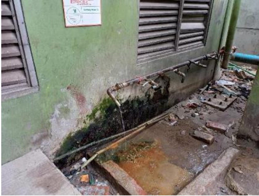
Dampness on wall and roof
