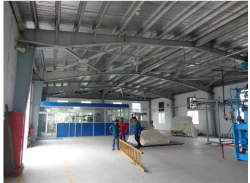
Lack of vertical load resisting system (bracing)
