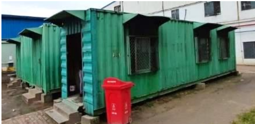
Lack ground anchorage and foundation system for ancillary 2 & 3 (Canteen & Smoke Shed)
