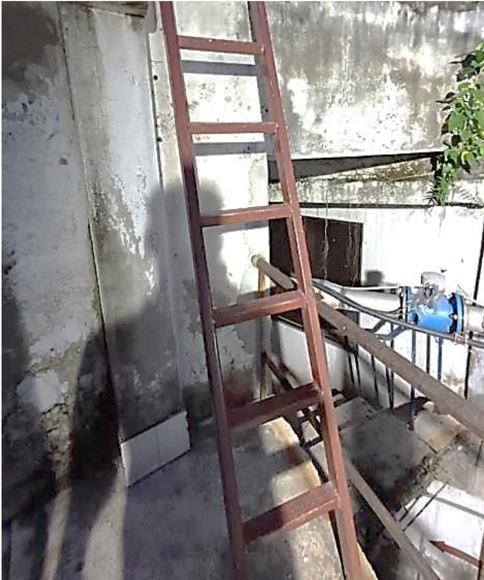
Dampness and vegetation on exterior wall
