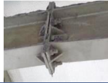
Gap between connection plates
