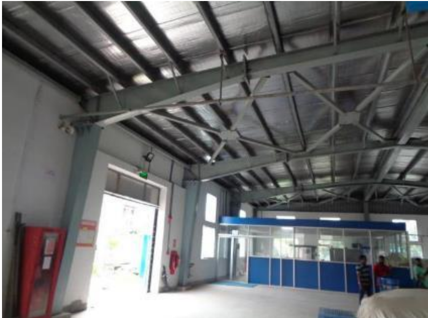
Lack of vertical load resisting system (bracing)
