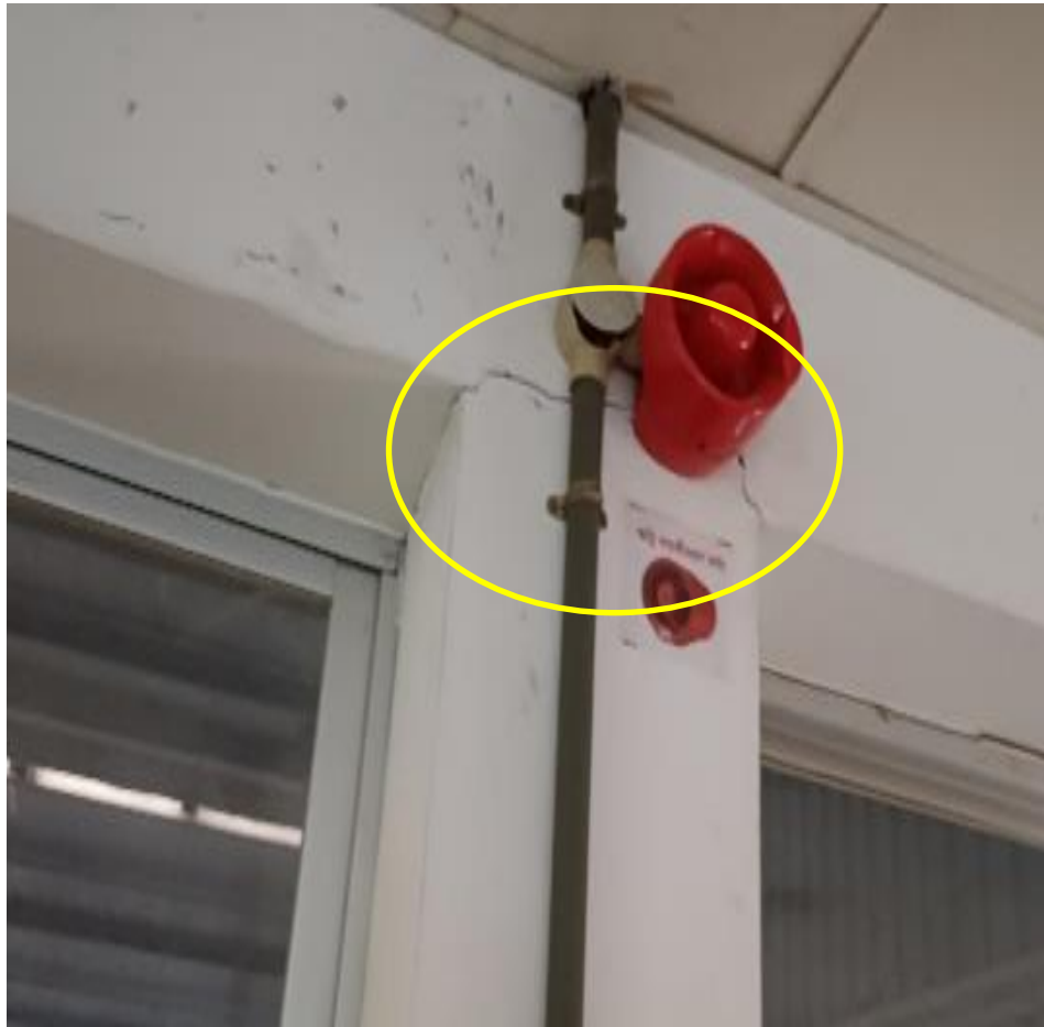
Crack on wall at several locations
