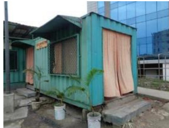
Lack ground anchorage and foundation system for ancillary 4, 5 & 6 (General Security Post, Female Security Post and Container Security Office at main gate)
