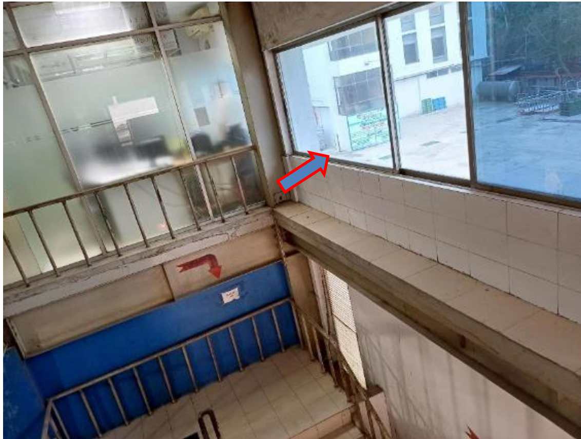
Falling hazard at mezzanine floor due to low height masonry wall
