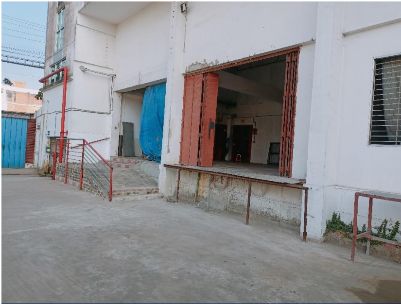
Column and beams adjacent of driveway of loading unloading zone
