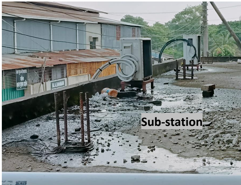
Exposed rebar on roof
