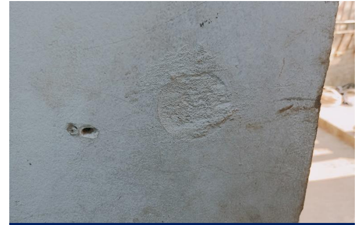
Core cutting location
