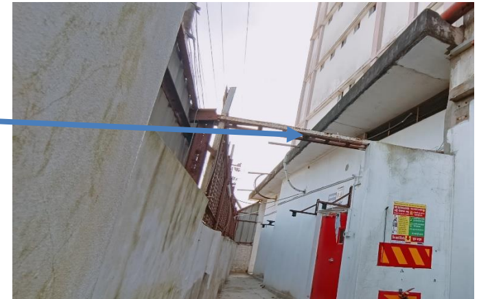
Slab of sub-station
