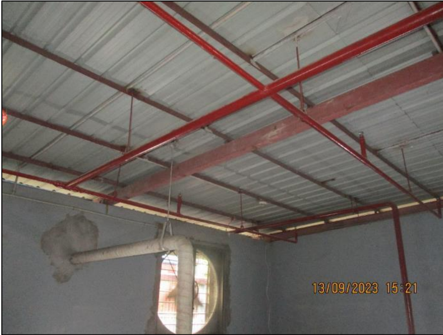
Light weight roof supported on peripheral wall
