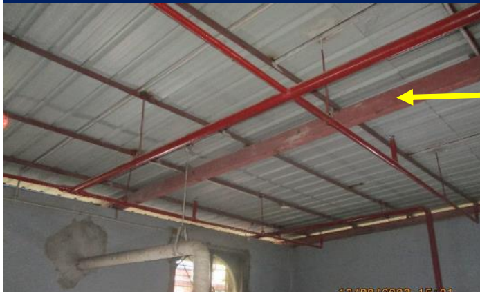
C-channel rafter at roof
