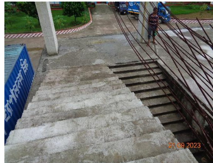
Missing railing at stair
