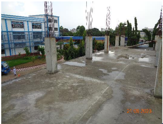
Parapet wall missing at roof
