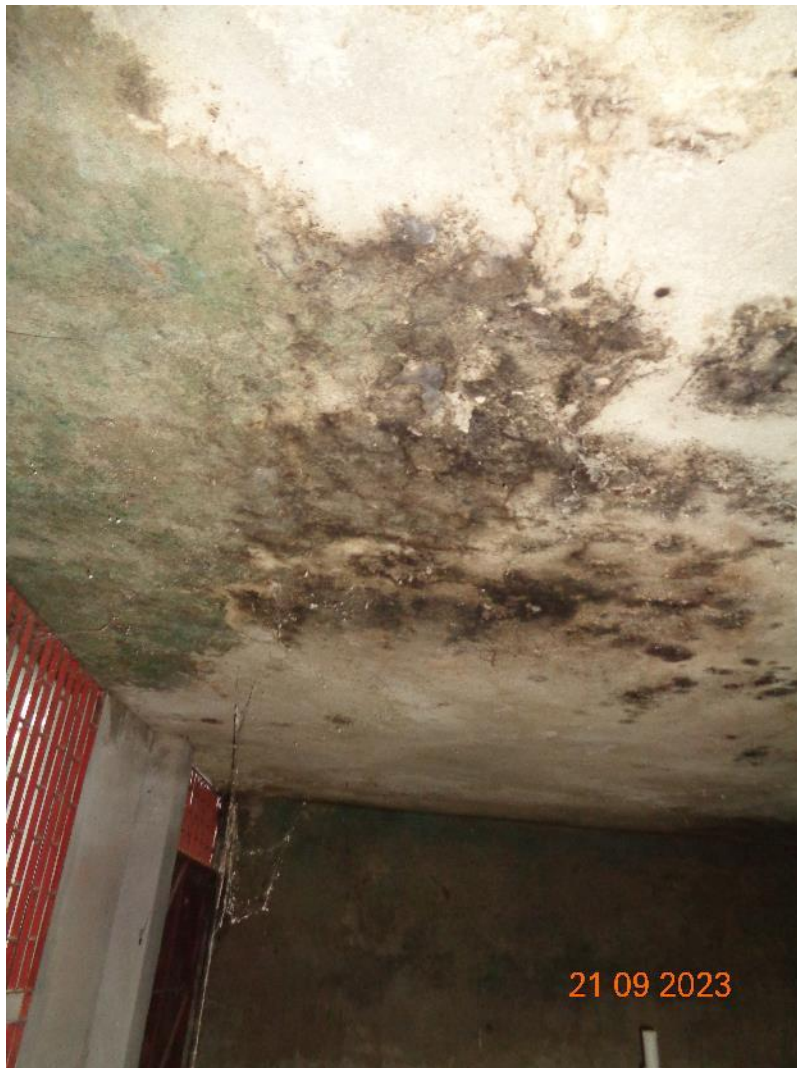
Dampness on Wall & slab
