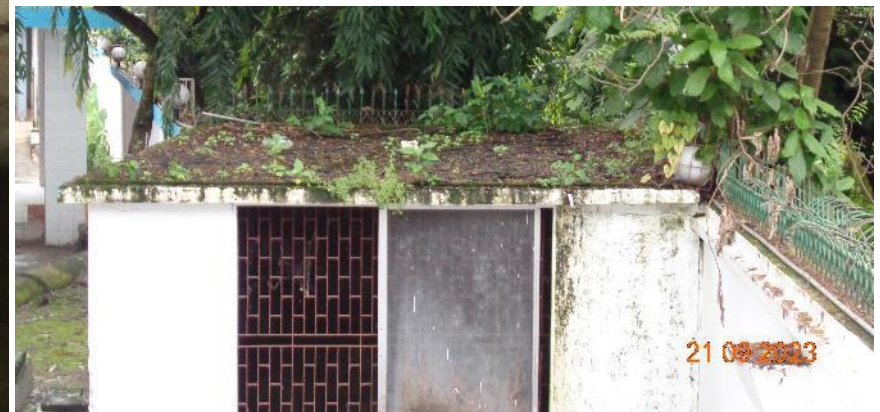
Dampness on Wall & slab
