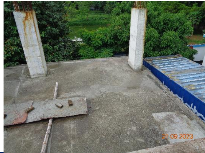
Parapet wall missing at roof
