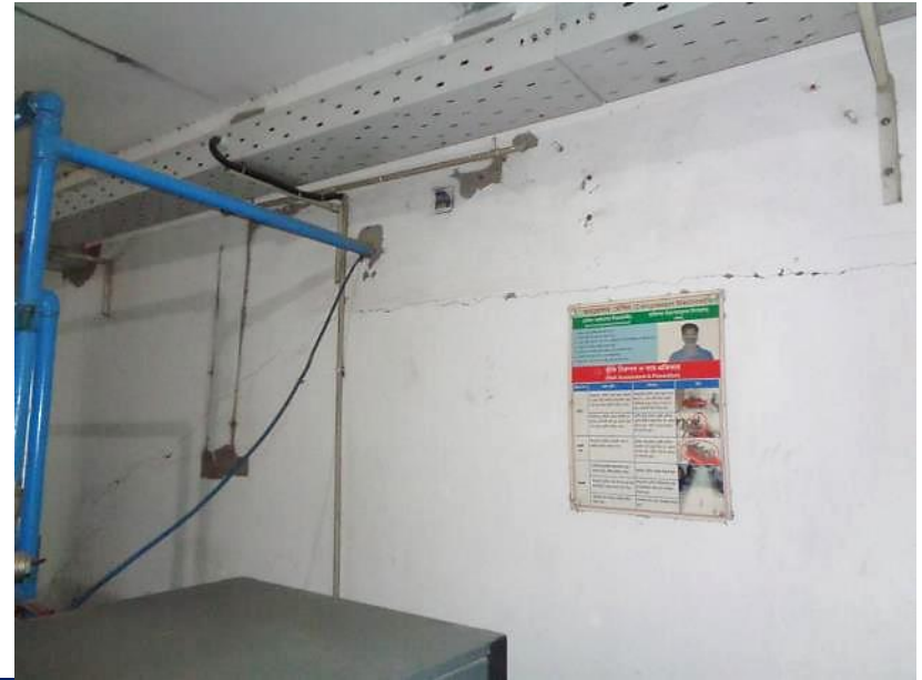
Crack in brick walls & floors
