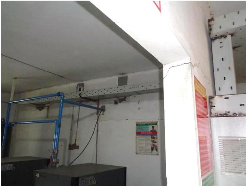
Crack in brick walls & floors
