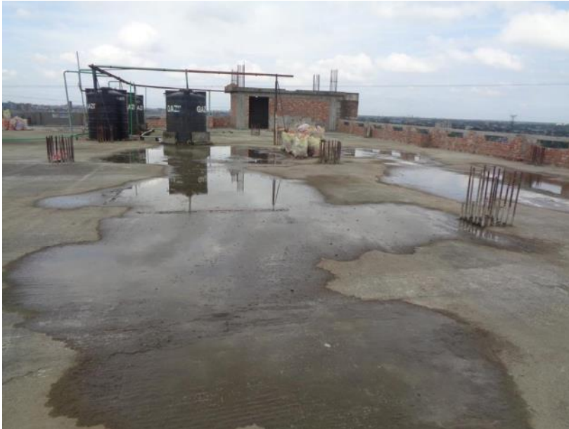
Water ponding on the roof
