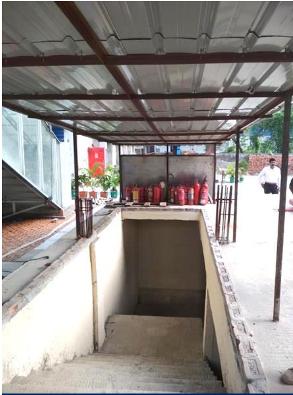
Lightweight steel shed above staircase
