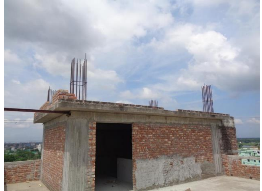
Exposed rebar on roof
