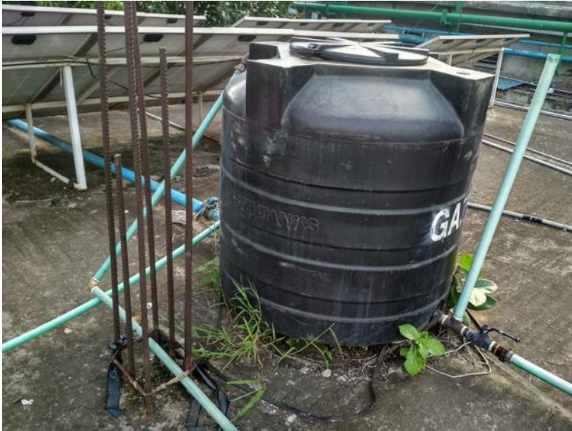
Exposed rebar on roof
