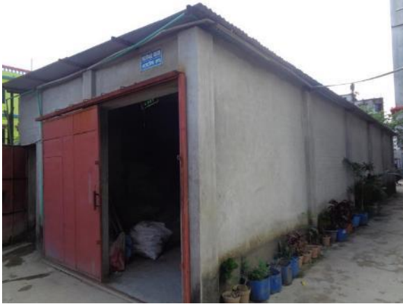
Peripheral brick walls
