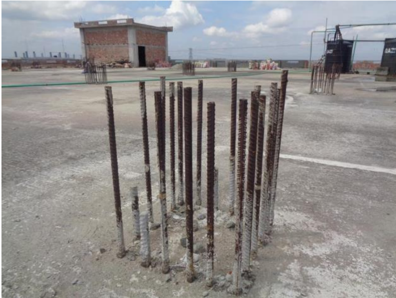
Exposed rebar on roof
