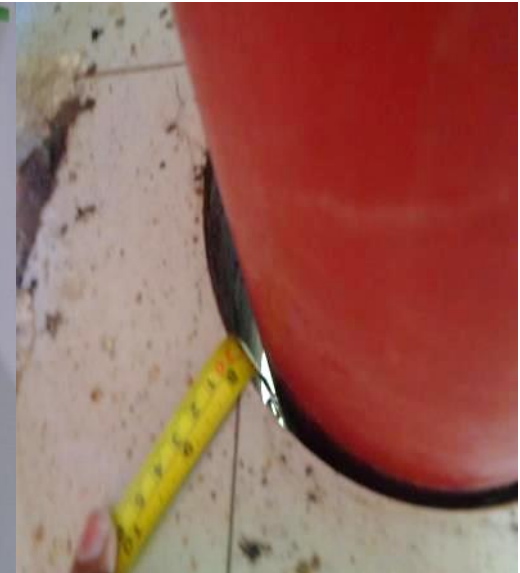
Stone chips aggregate in Main Building as per test report and floor slab punch.
