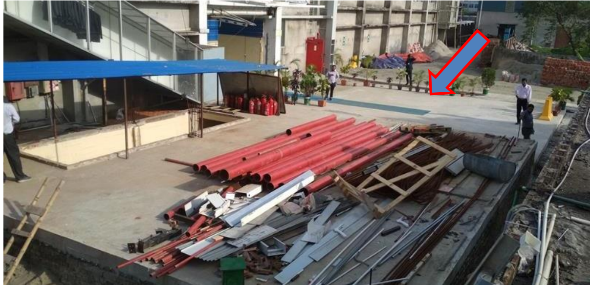
Roof of fire pump room used for loading unloading zone
