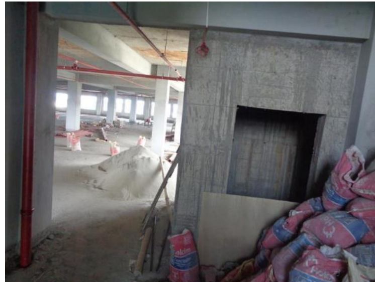
Onsite: Shear wall in lift core
