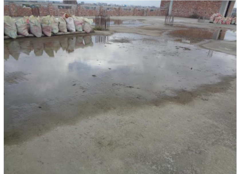
Water ponding on the roof
