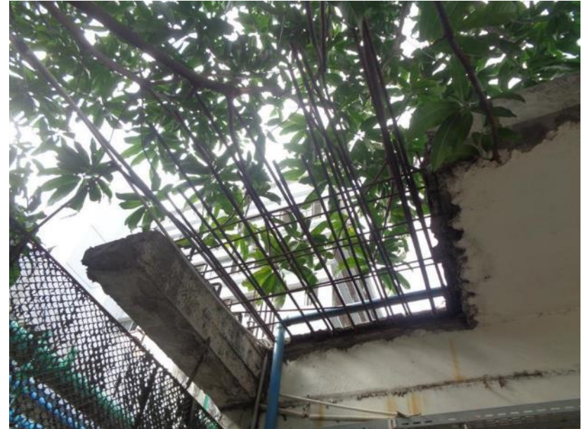
Exposed rebar on roof
