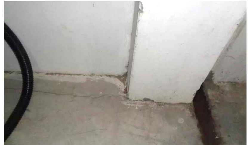
Crack in brick walls & floors
