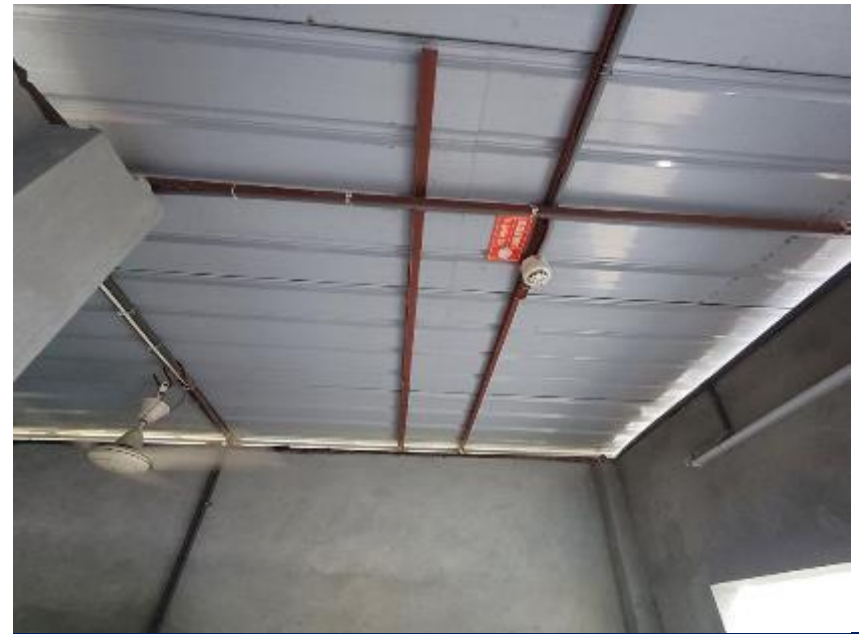
Steel angel connection with wall
