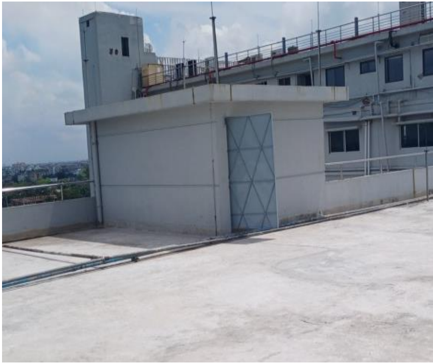
Rooftop staircase slab rested on brick wall
