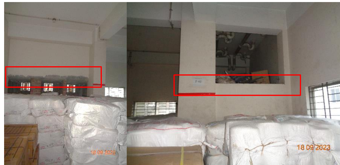
False slab in toilet zone area
