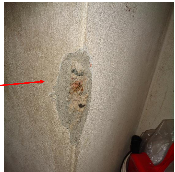
Stone chips Aggregate in column
