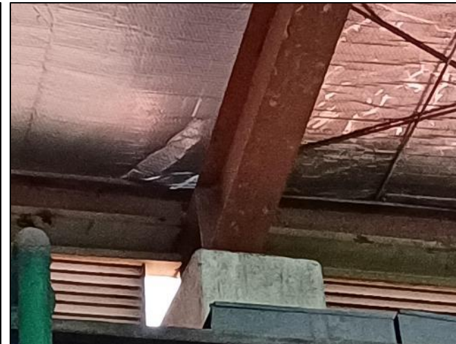
Connection of rafter with RC column
