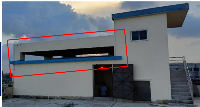
Additional slab at the roof of the stair top
