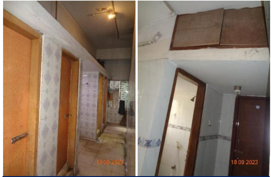
False slab in toilet zone area
